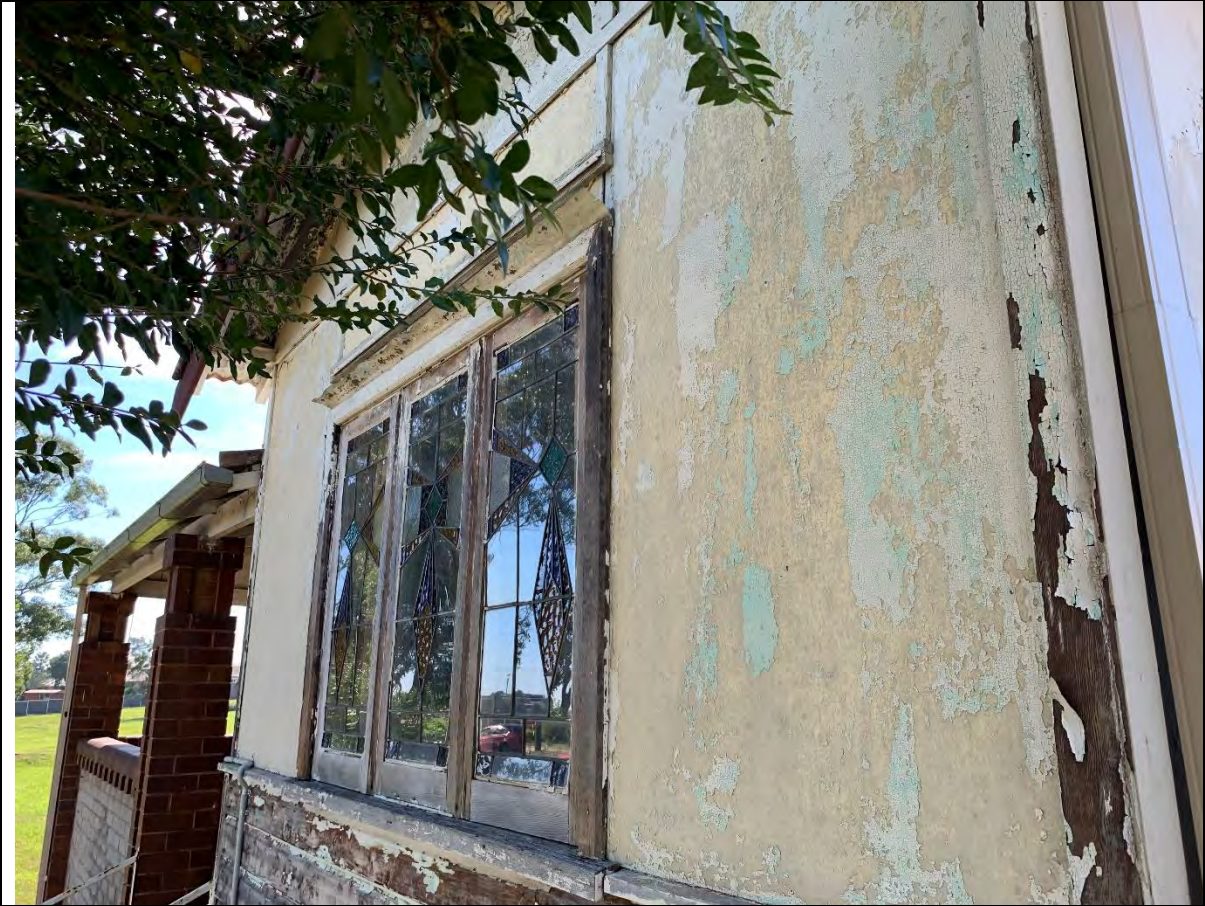
Photo 6 -View to the north showing the western face of the residence. The windows are stained glass and the comes (parts holding glass together) are presumably composed of lead.
