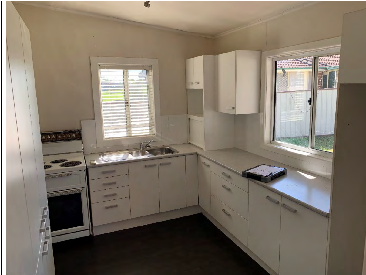
Photo 15 - View to the north showing the kitchen (Room 2). The western wall (exposed and beneath particle board) in this room is presumed to be composed of non-friable ACM sheeting. The other walls are covered with ceramic tile and wood particle board painted with lead-based paint.
