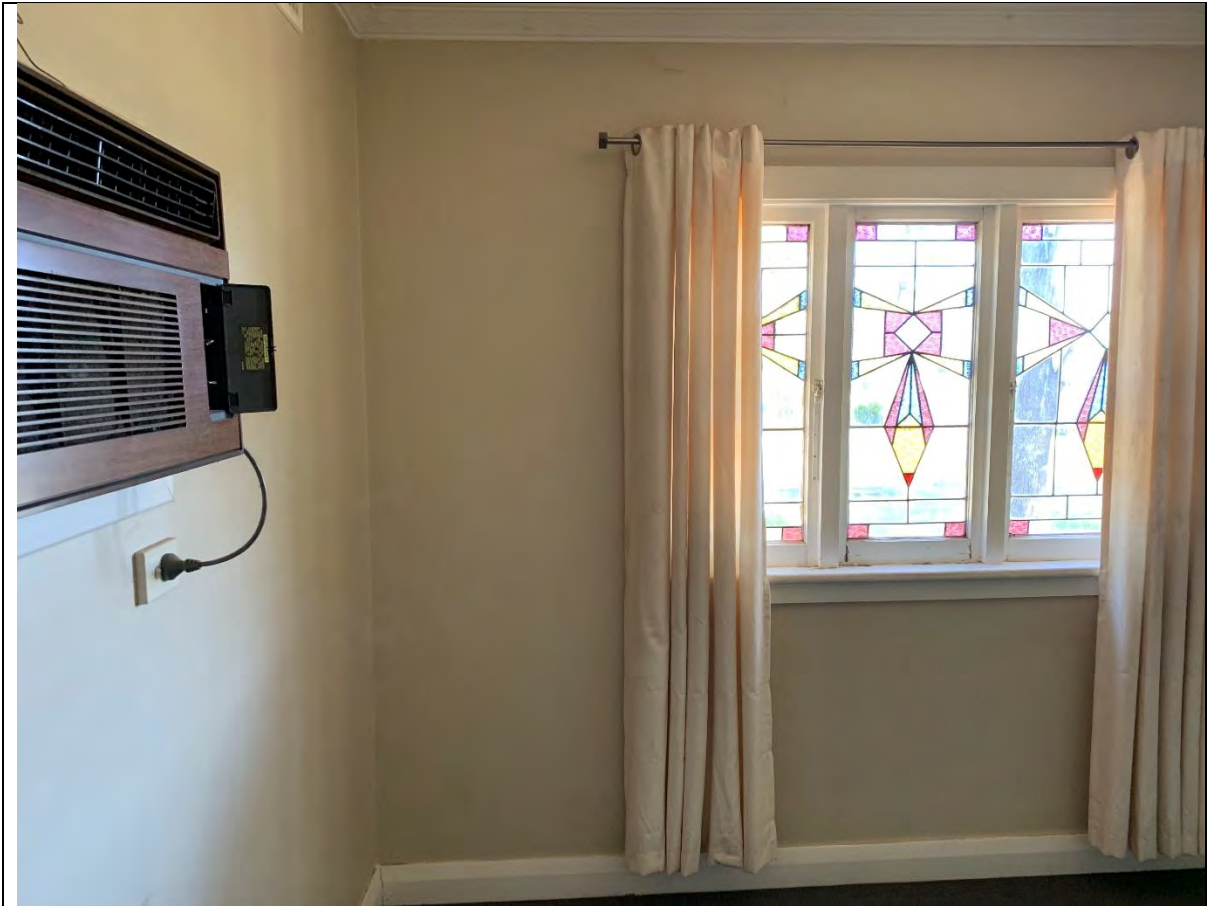
Photo 25 - View towards the west showing a stained-glass window in Room # 7. The comes (material holding glass together) are presumably composed of lead.
