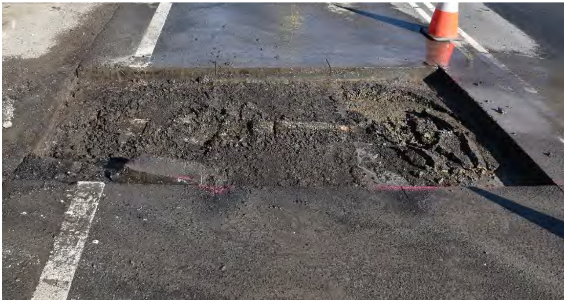
Figure 4-2: Test trench 1 showing top of context 05 – bituminous asphalt
