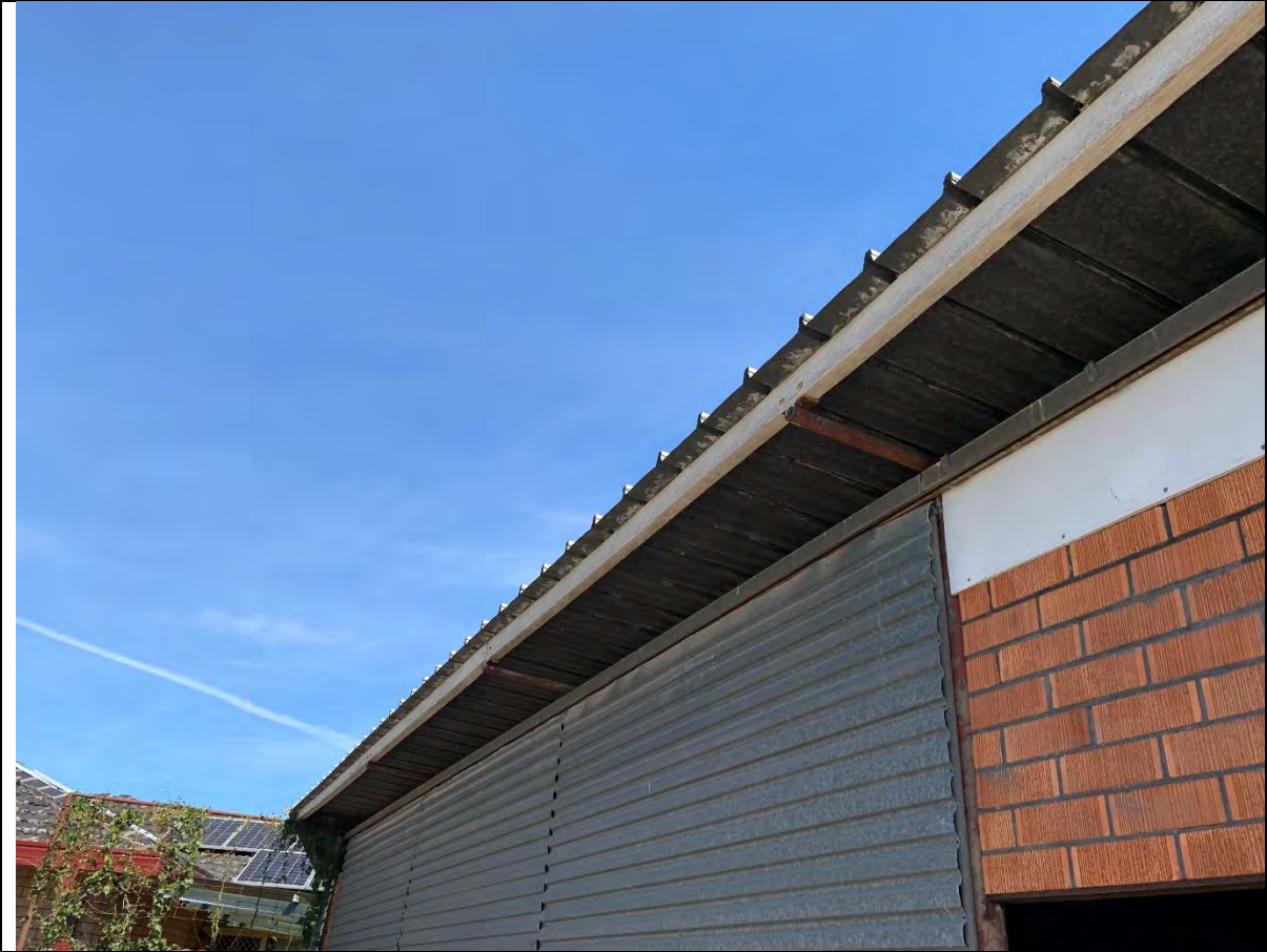
Photo 31 - View to the south showing Garage # 1. The fascia trim contains wood covered with white lead-based paint
