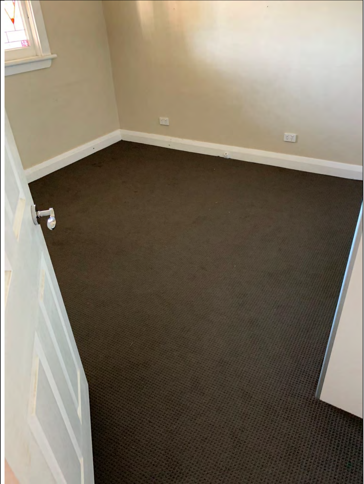
Photo 24 - View towards the southwest showing the carpet in the bedroom (Room # 6).
