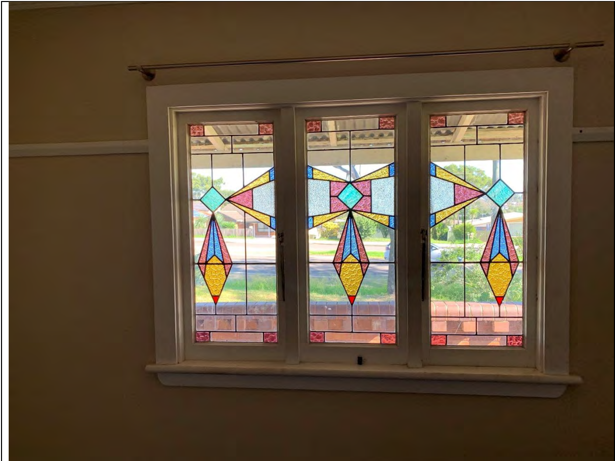
Photo 23 - View towards the west showing a stained-glass window in Room # 6. The comes (material holding glass together) are presumably composed of lead.
