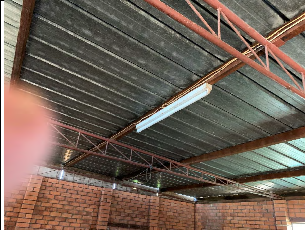
Photo 34 - View of the ceiling of Garage # 1 showing a fluorescent light.
