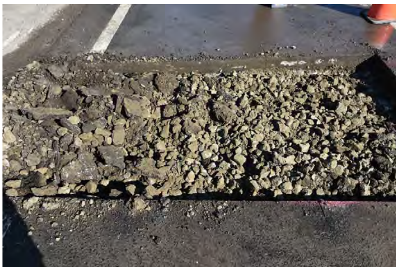
Figure 4-4: Test trench 1 showing interface at base of context 02 (basalt ballast) and the top of context 03 (ironstone ballast) and attempts to excavate by hand
