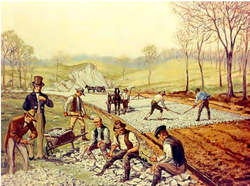
Figure 2-1: 1823-First American Macadam Road (painting by Carl Rakeman - from U.S Department of Transportation)
