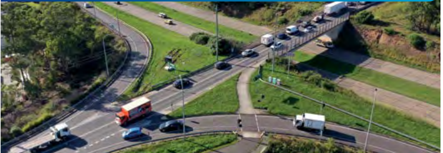
Prospect Highway looking south towards M4 Motorway
