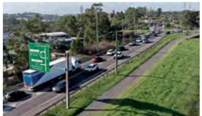
Prospect Highway looking south towards M4 Motorway
