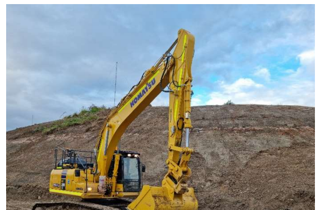
Above: Excavations works between M4 Motorway and Reservoir Road ongoing.
