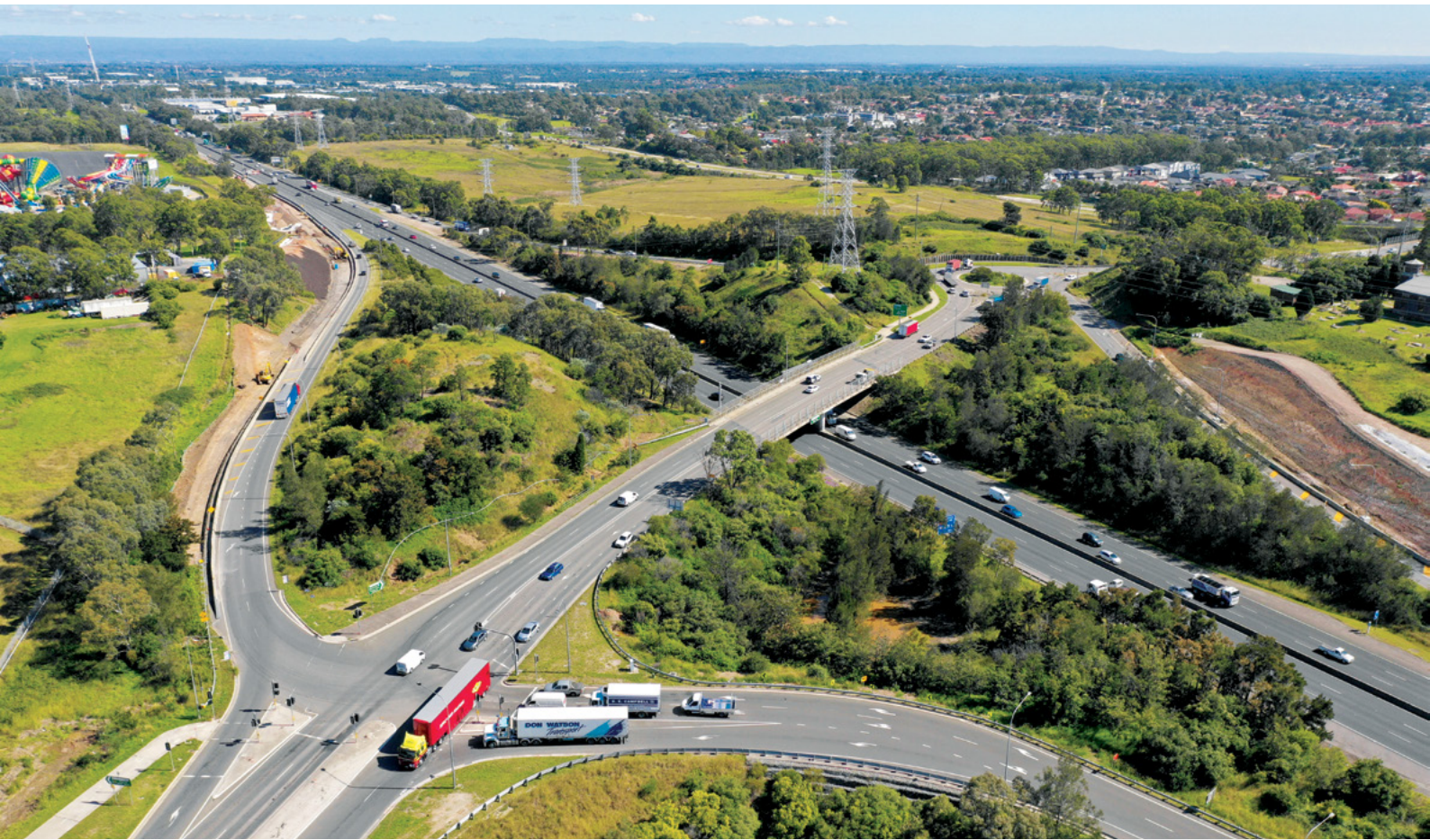
Prospect Highway and M4 Motorway interchange looking north west
