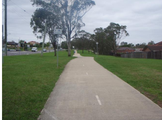
Photo A2, shared user path western side of Prospect Highway, towards south
