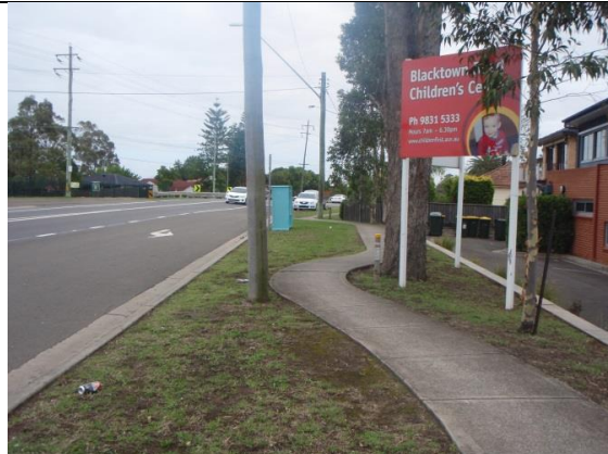
Photo A6, concrete footpath adjacent to Blacktown Road Children's Centre, towards north
