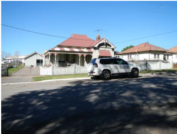
Plate 12: 'Bridestowe' house, view to south-east across Reservoir Road.
