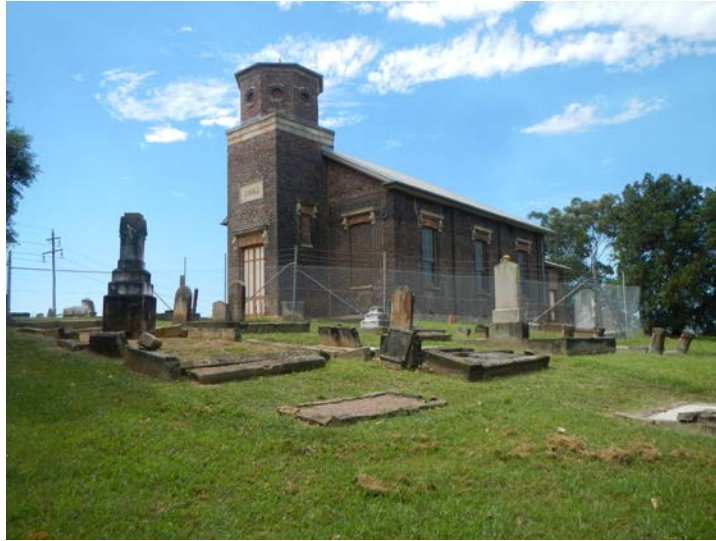
Plate 6: St Bartholomew's Church
