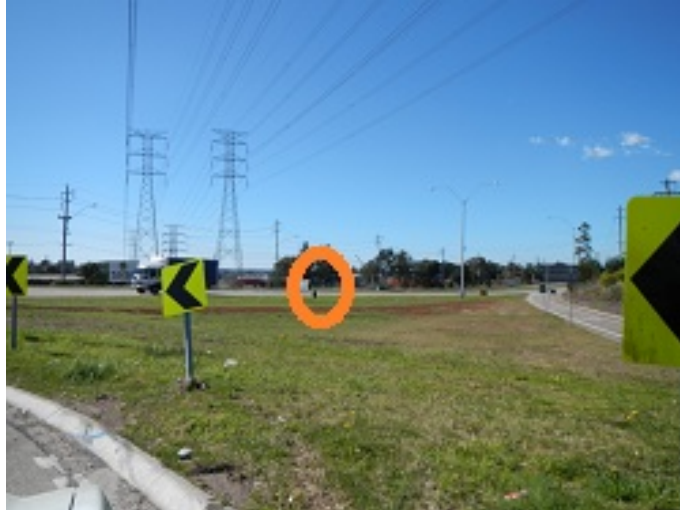
Photo 6-7 Milestone (circled orange) along southern edge of the Great Western Highway, view to north-east (taken from Ponds Road)
