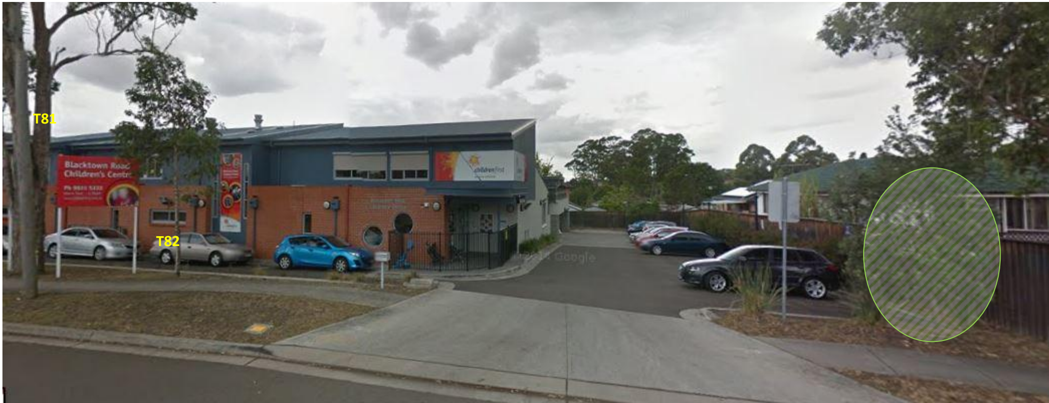
Image 28: Blacktown Child Care Centre, 217-221 Blacktown Road, southern corner.
