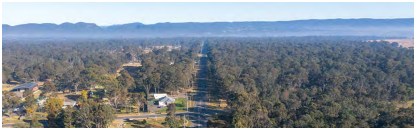
Aerial view of Londonderry Road and The Driftway
