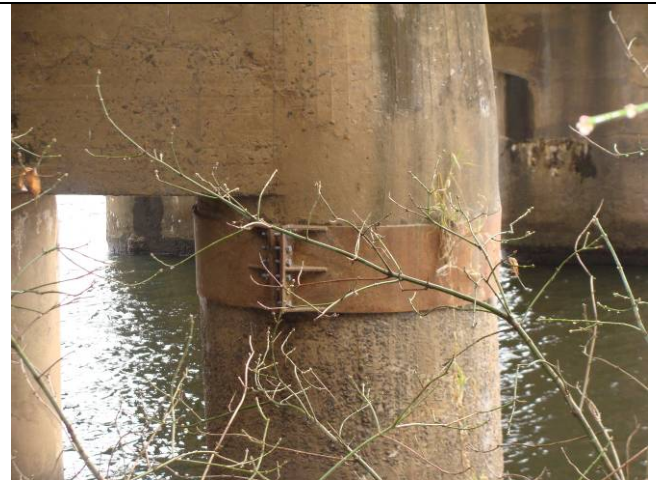
Photo 34-(B-43)Span 4 Pier 4 column 1 Upstream crack at joint
