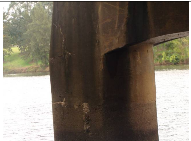
Photo 34-(B-43)Span 4 Pier 4 column 1 Upstream crack at joint
