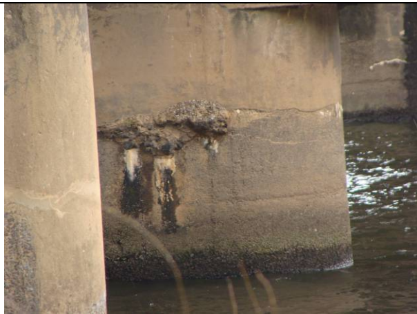
Photo 33– (B-40)Span 5 Pier 5 & Pier 6 column2 - crack at pier construction joint
