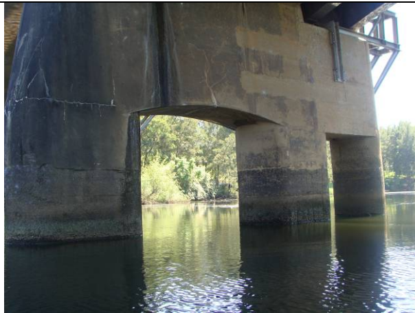
Photo 33– (B-40)Span 5 Pier 5 & Pier 6 column2 - crack at pier construction joint
