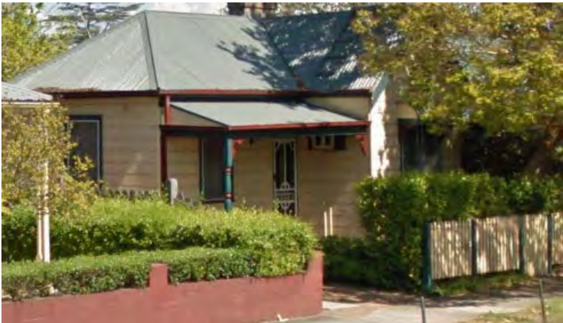
Figure 6-13b House, 160 March Street (Item I482)
