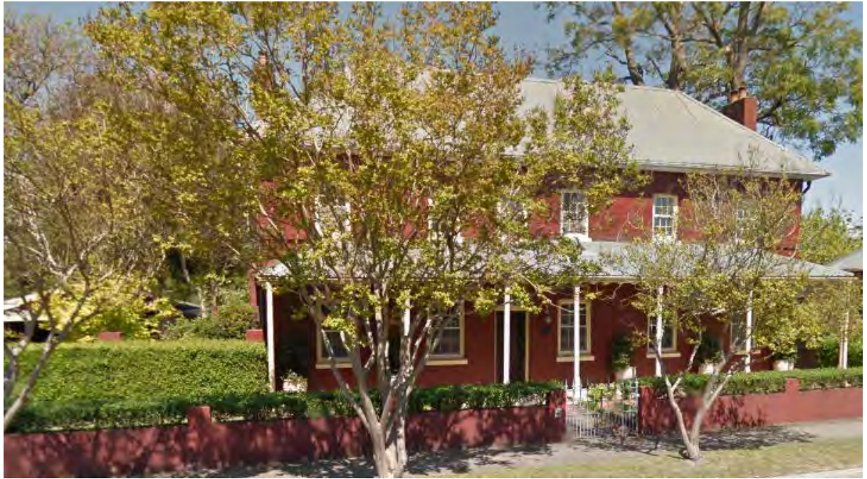
Figure 6-14 Rutherglen – 158 March Street (Item I69)
