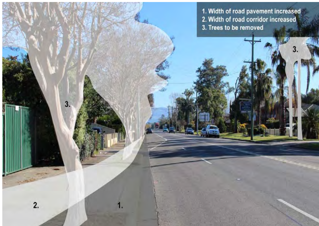
Figure 6-6 Indicative extent of proposed work along March Street (west of the Bosworth Street intersection) as viewed from the Bosworth Street intersection
