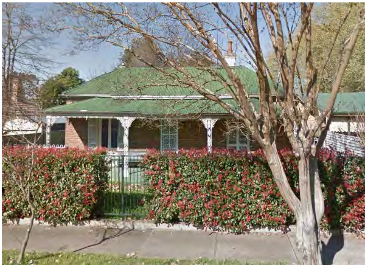
Figure 6-10 House, 190 March Street (Item I72)
