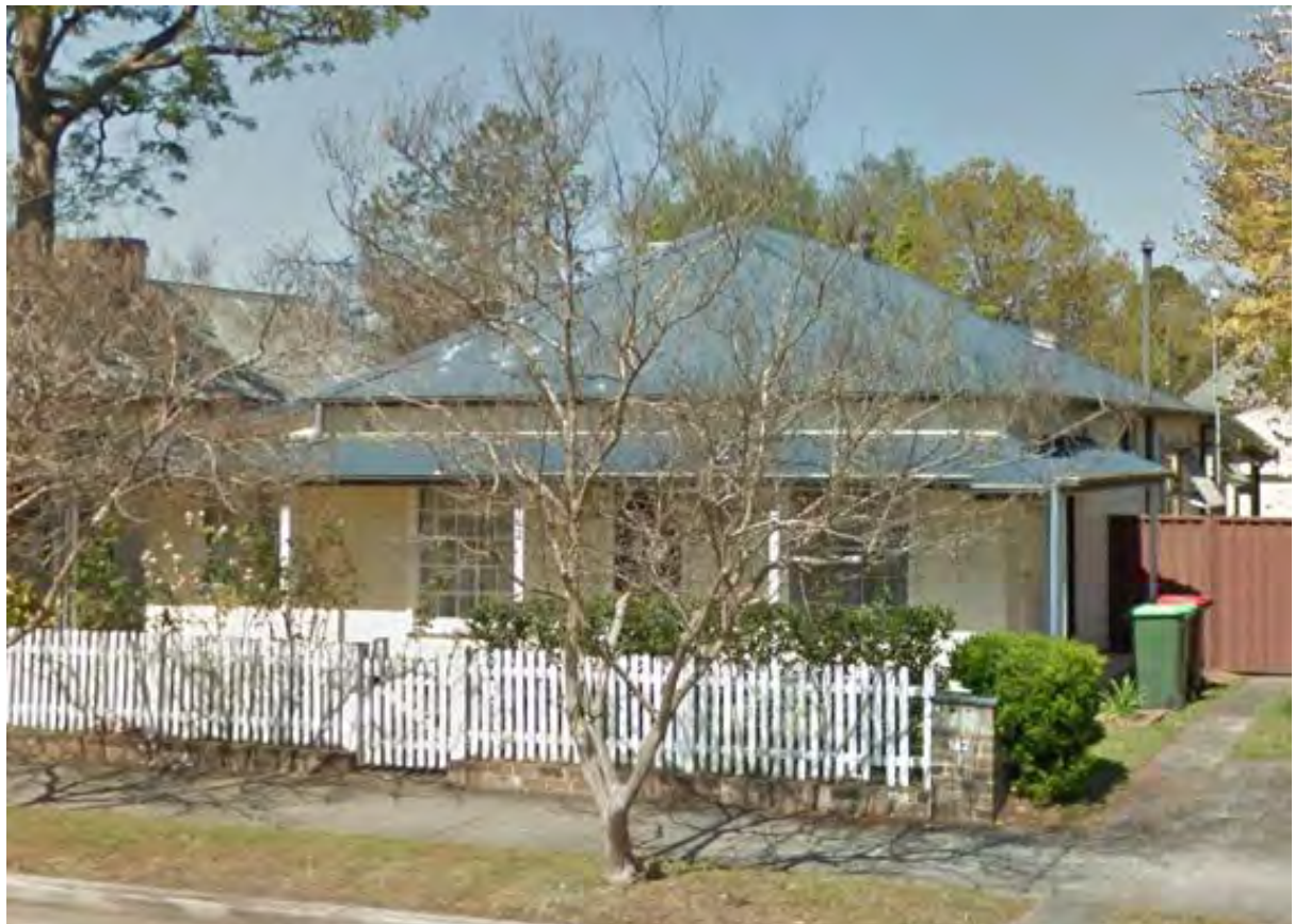
Figure 6-12 House, 162 March Street (Item I483)
