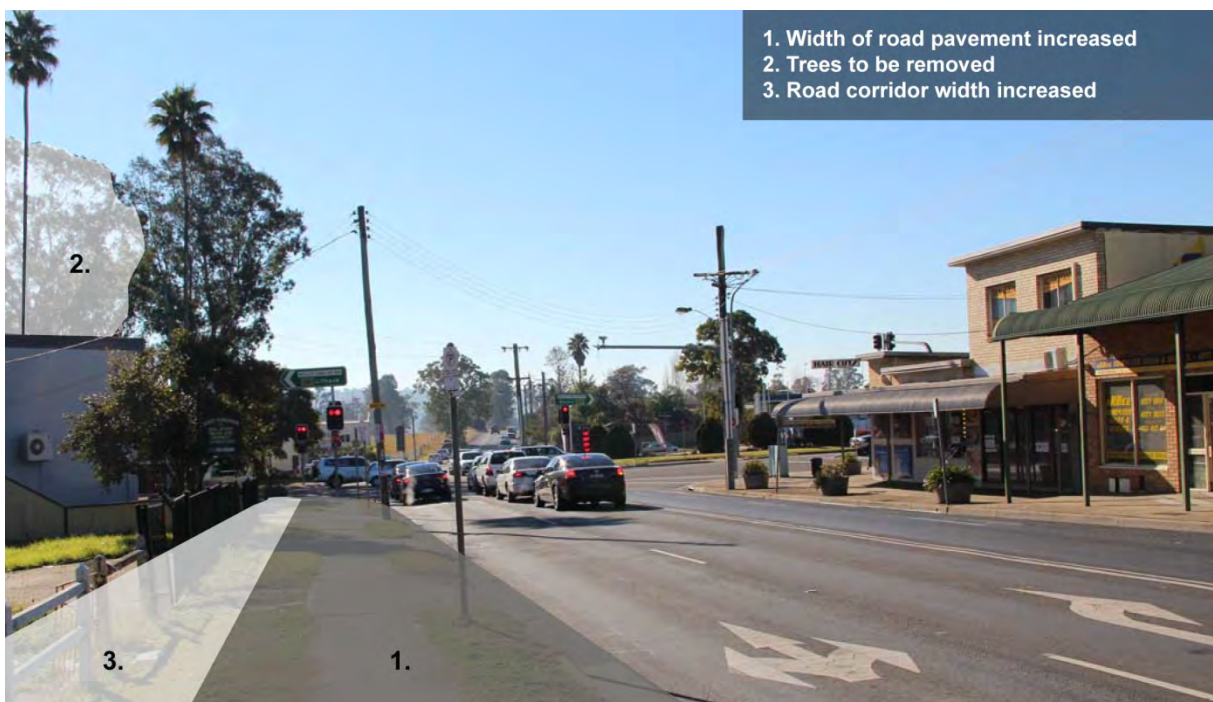
Figure 5 - The proposed works as views from the Grose Vale Road northbound approach to the intersection
