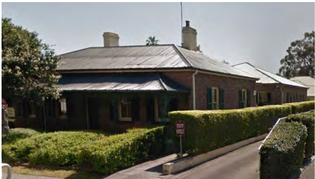
Figure 6-15 House, 155 March Street (Item I71)
