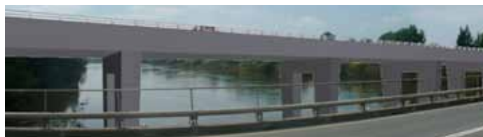
View from shared path looking downstream at new bridge.
