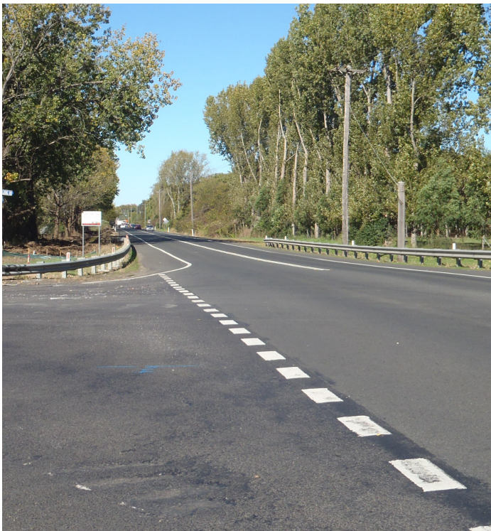
Intersection of Kurrajong Road and Old Kurrajong Road, Richmond
