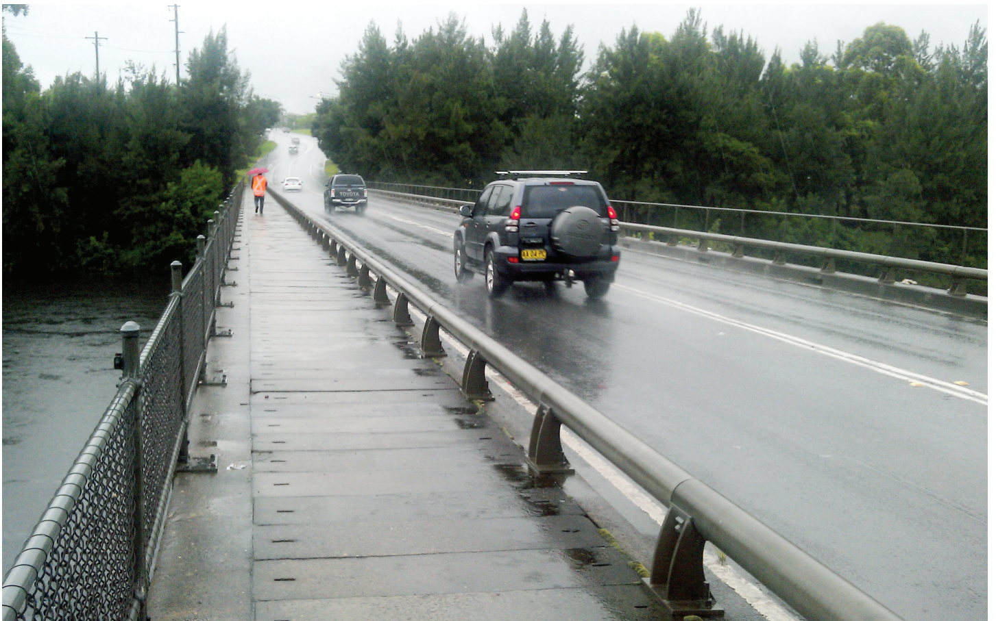
Richmond Bridge looking westward towards North Richmond
