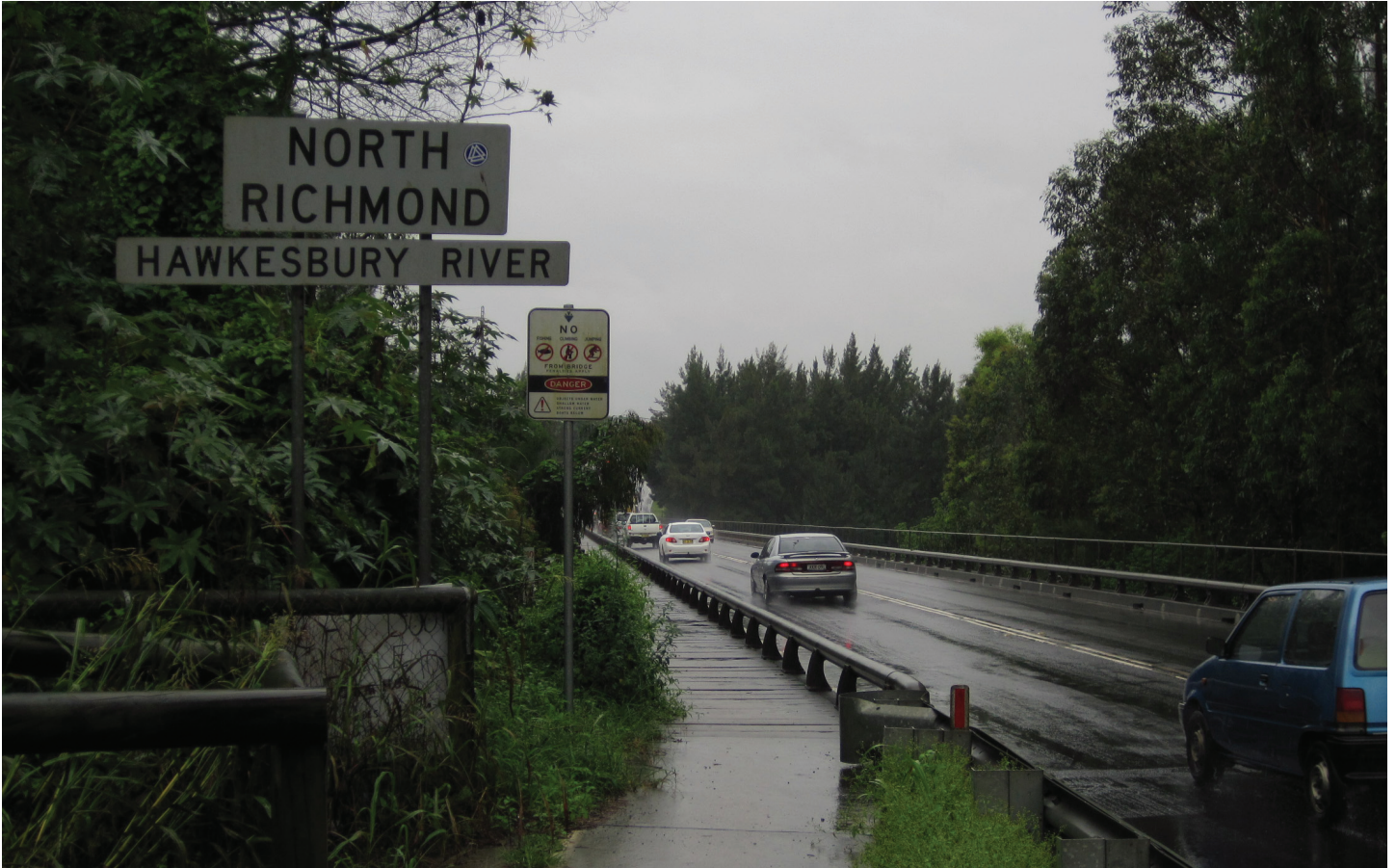
Richmond Bridge looking toward North Richmond
