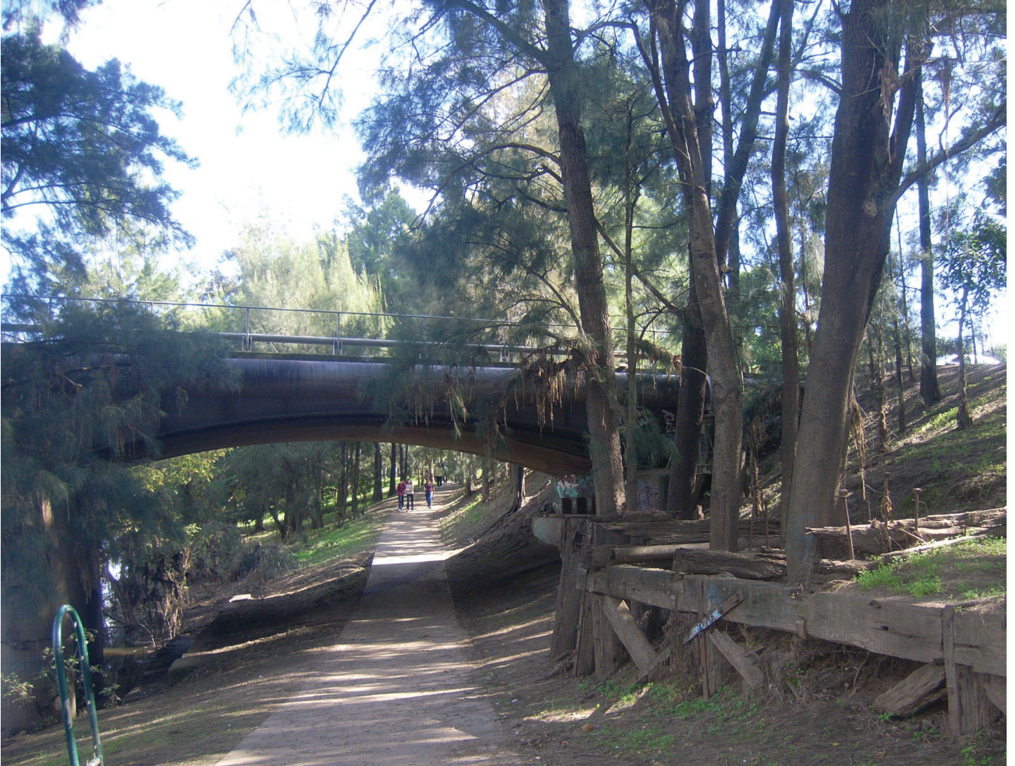
Richmond Bridge pedestrian underpass adjacent to Hanna Park
