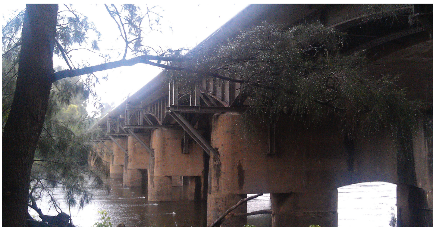
Downstream side of Richmond Bridge
