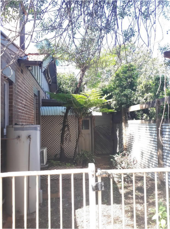
Figure 12: Shed along southern boundary of the item (Courtesy: Hutchison Weller).
