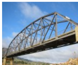
h00989 bethanga bridge bellbridge pratt truss north nsw 01 jun20044 mz
