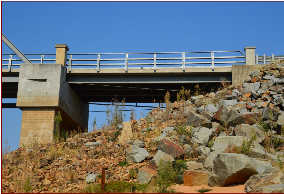
Plate 1: Additional span added to the NSW side of the bridge in 1963
