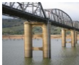
h00989 bethanga bridge bellbridge pylons 01 jun20044 mz
