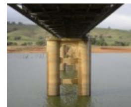
h00989 bethanga bridge bellbridge pylons 02 jun20044 mz
