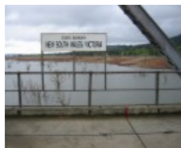
h00989 bethanga bridge bellbridge border jun20044 mz
