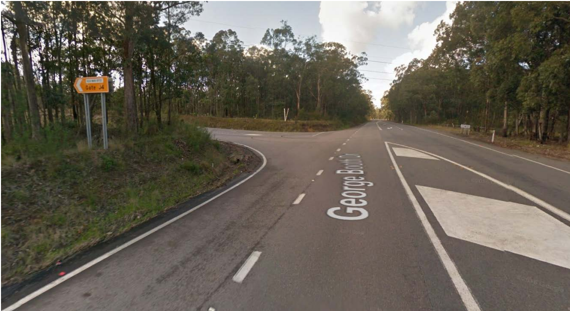
Figure 2.2 : George Booth Drive facing eastbound direction towards the site access
