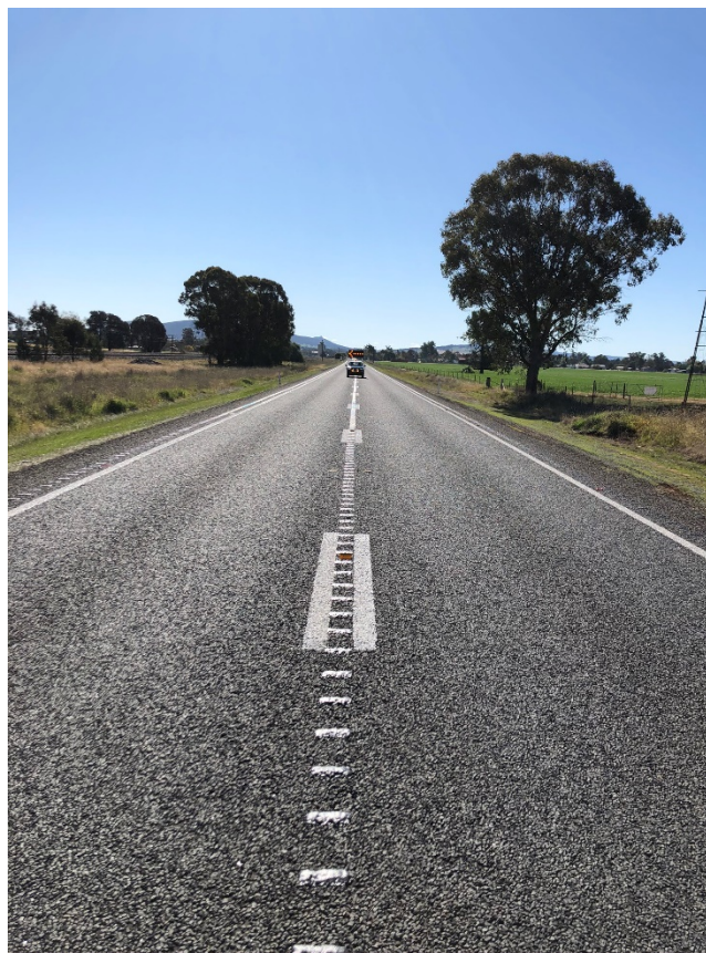
Rumble strips being installed.
