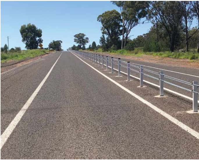
Wide centreline and barriers installed in section three.
