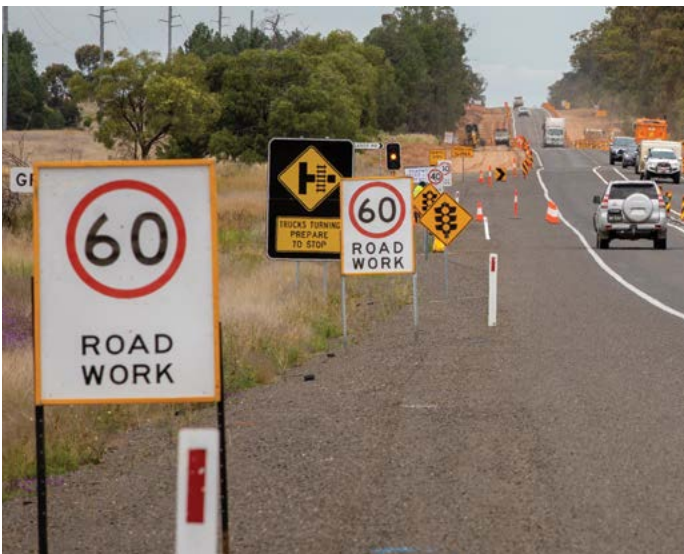
Work in progress on section two.
