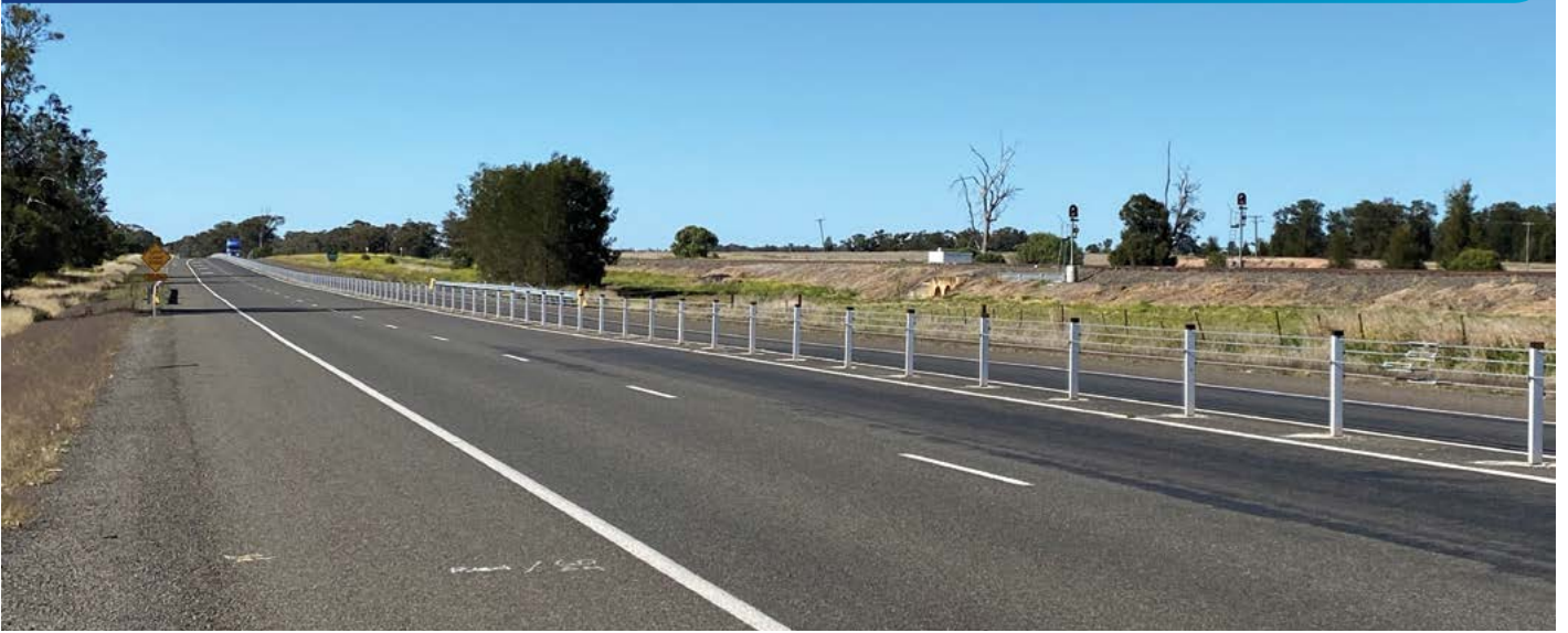
Section one of the project is complete.
