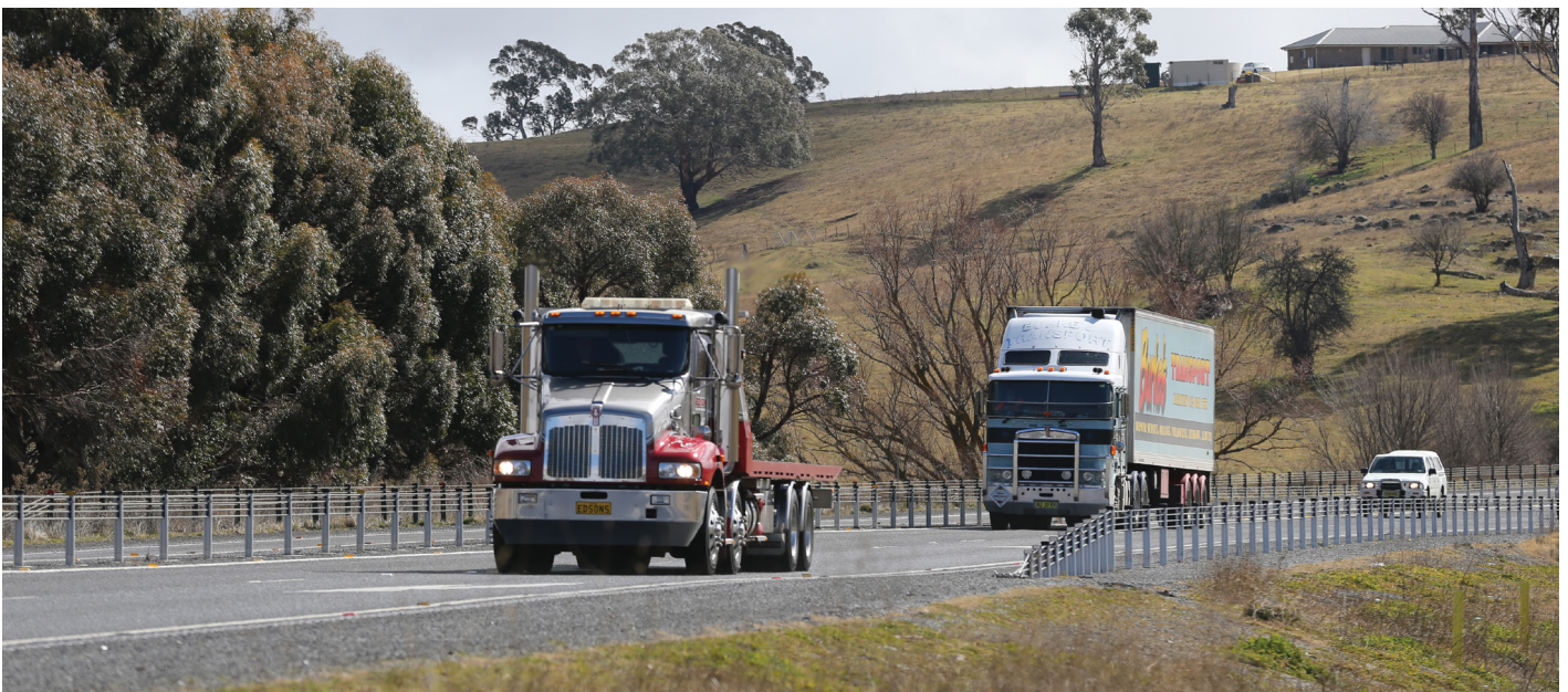
Flexible safety barrier installed in the centre median and roadside at East Lucknow on the Mitchell Highway
