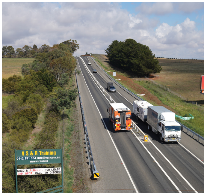
Mitchell Highway flexible safety barrier treatment at Oak Creek Lane
