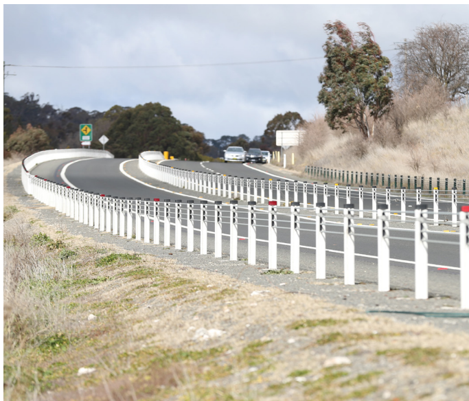
Mitchell Highway flexible safety barrier treatment at East Lucknow
