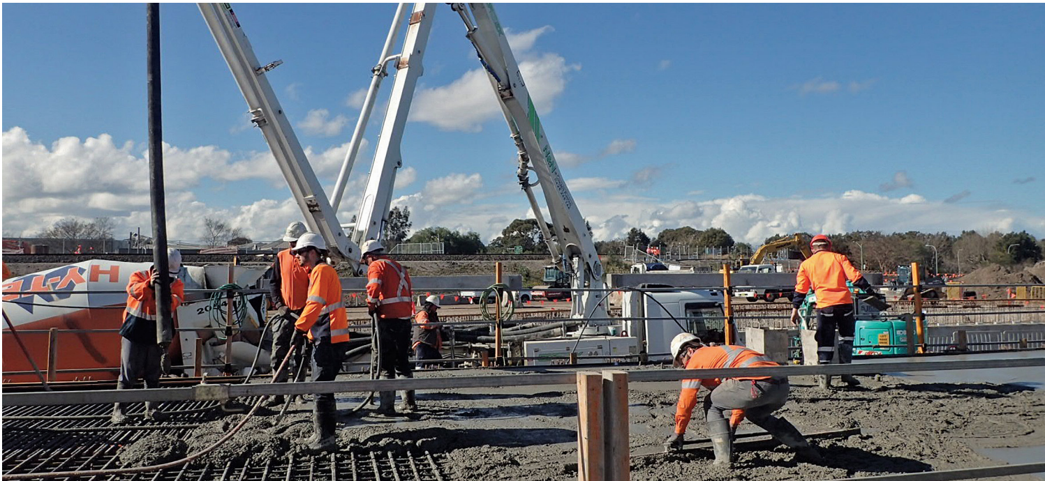
Canal Bridge under construction
