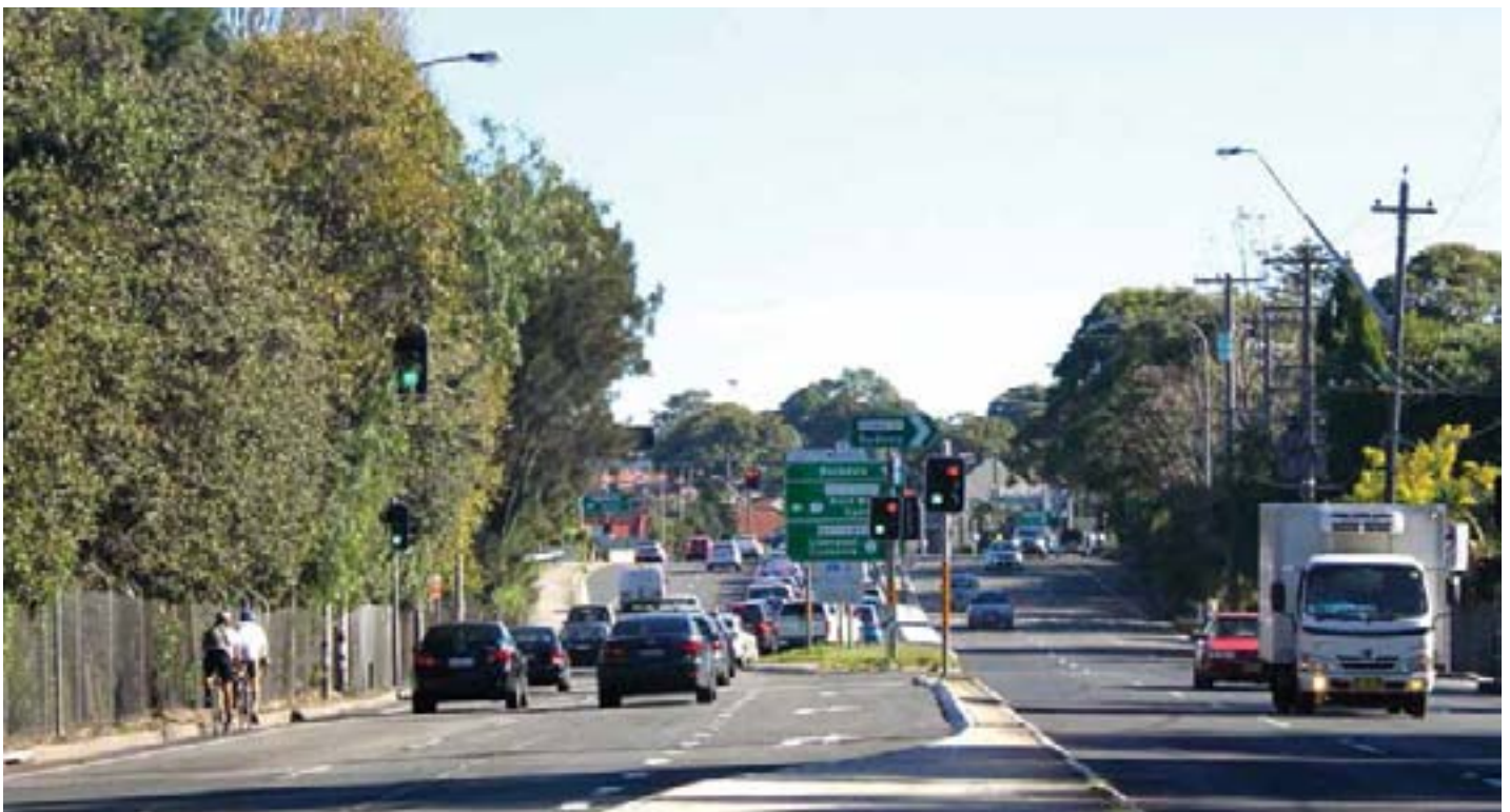
Existing Marsh Street looking west
