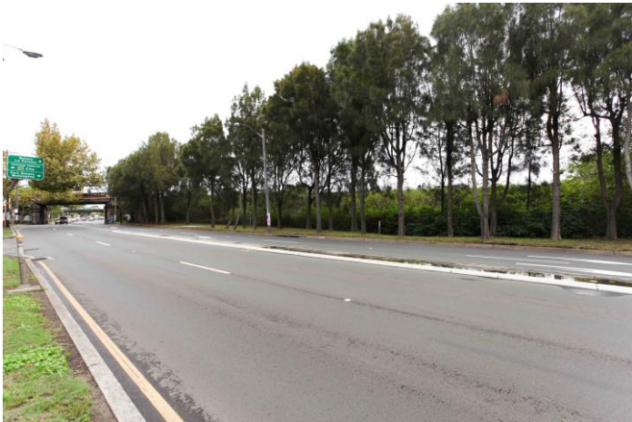
Image 5.23. Sheoaks along the west side of Botany Road north of Bronti Street. Stedinger Associates 2014. Image 1692.
