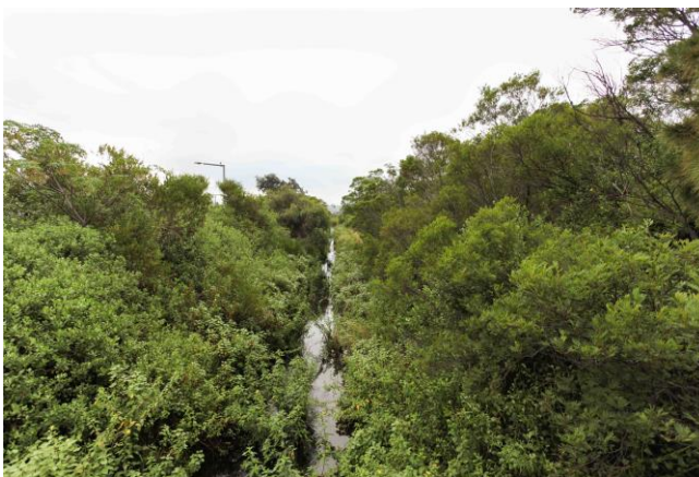
Image 5.5. Drainage channel along General Holmes Drive. Facing north. Stedinger Associates 2014. Image 1728.
