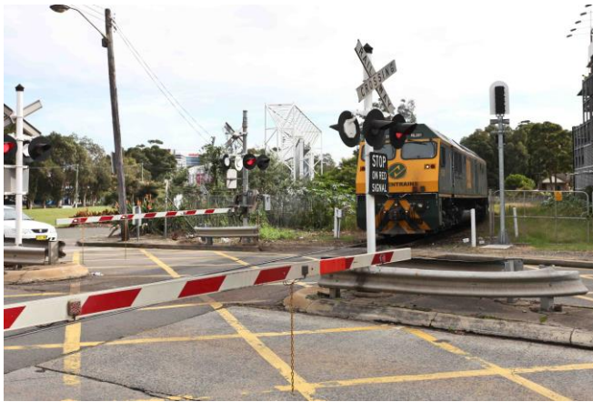
Image 5.7. The level crossing associated with the single Botany Line at General Holmes Drive and Botany Road. Facing north. Stedinger Associates 2014. Image 2125.
