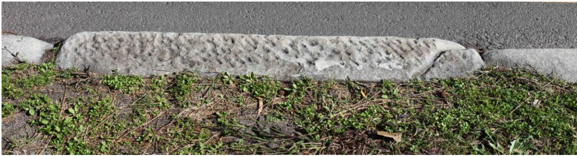
Image 5.20. Detail of pick marks in the sandstone kerbing. Facing west. Stedinger Associates 2014. Image 2154.
