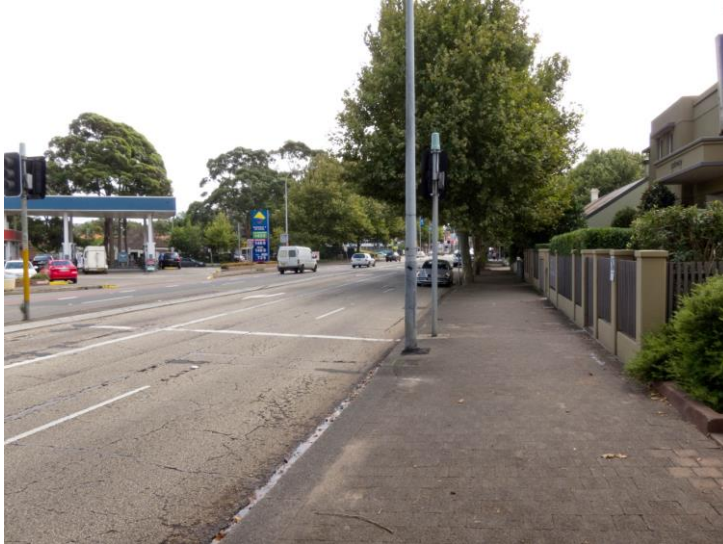
Image 5.17. Possible tram tracks, Plane trees and cottages beyond modern units along Botany Road (No.1247-1251). Facing north. Stedinger Associates 2012. Image 0352.
