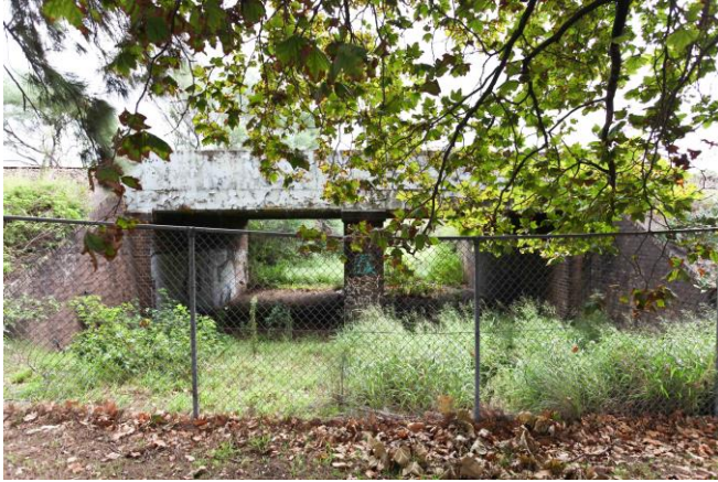
Image 5.10. Underpass beneath the railway embankment. Facing west. Stedinger Associates 2014. Image 1664.
