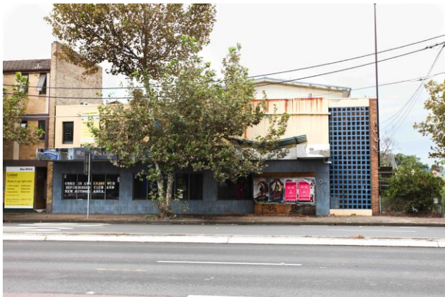
Image 5.2. Flats and offices along Botany Road, facing east. Stedinger Associates 2014. Image 1659.
