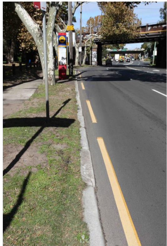
Image 5.19. An extensive line of sandstone kerbing between Bronti Street and the Mascot (Botany Road) Underbridge. Facing south. Stedinger Associates 2014. Image 2153.
