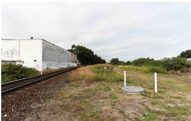
Image 5.8. The railway embankment along the Botany line. Facing south. Stedinger Associates 2014. Image 2119.
