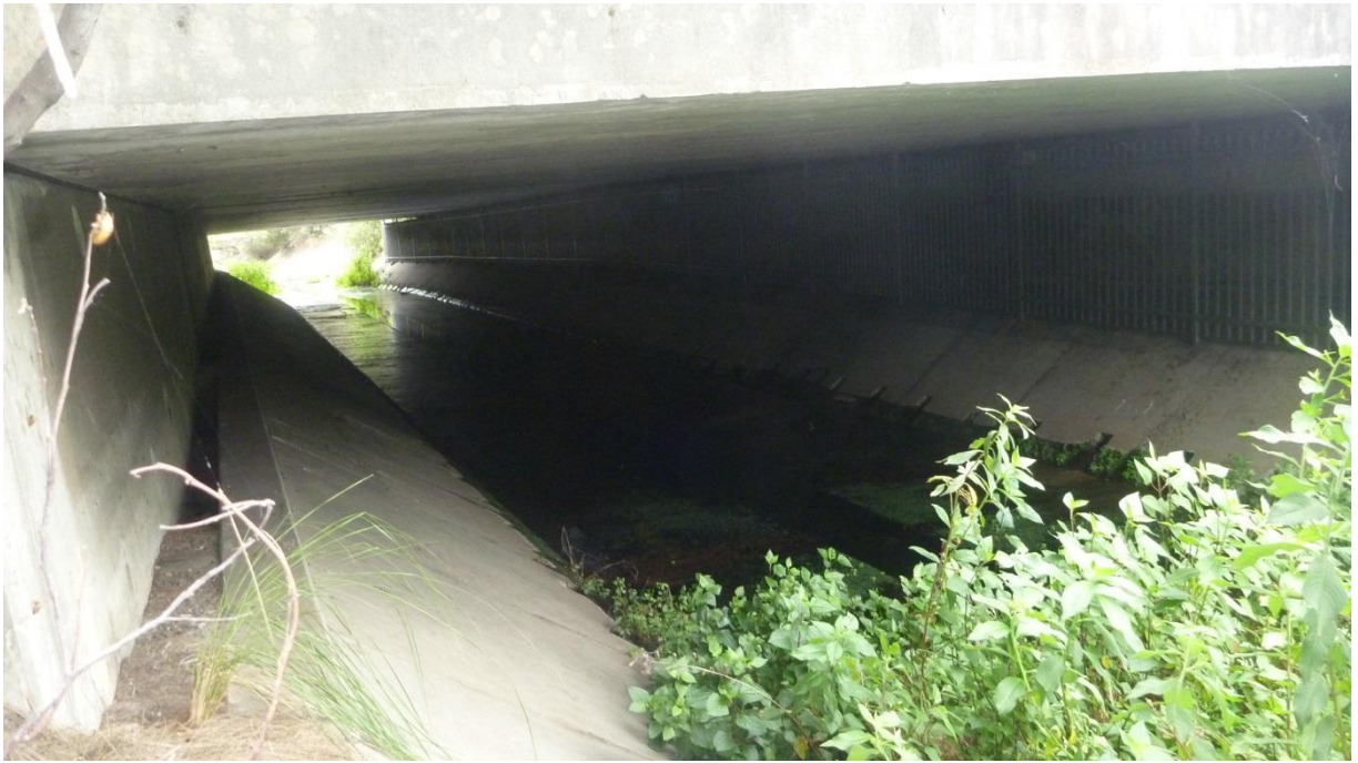
Plate 4.5 Existing Crossing Over Stormwater Channel at Mill Pond Road
