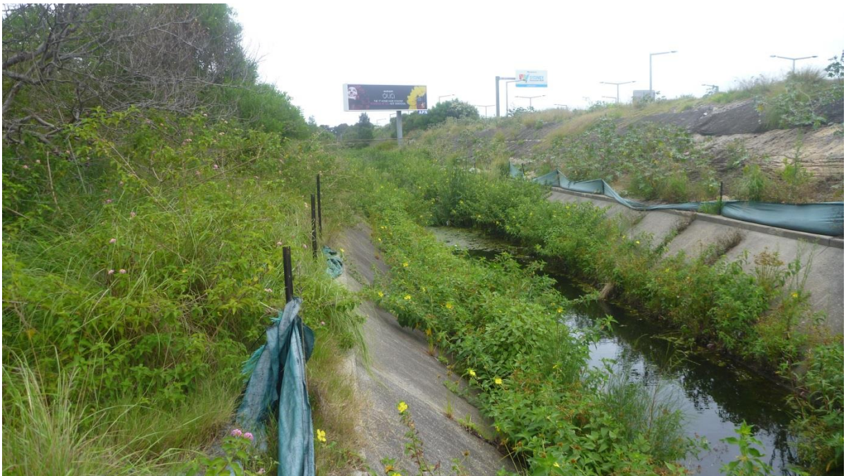
Plate 4.6 Existing Stormwater Channel Looking Downstream From Discharge Culvert
