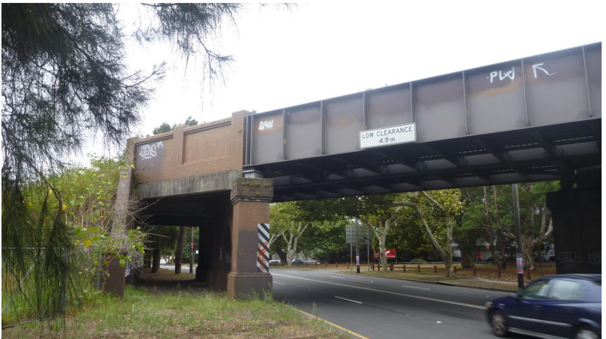
Plate 4.4 Existing Railway Overpass of Botany Road
