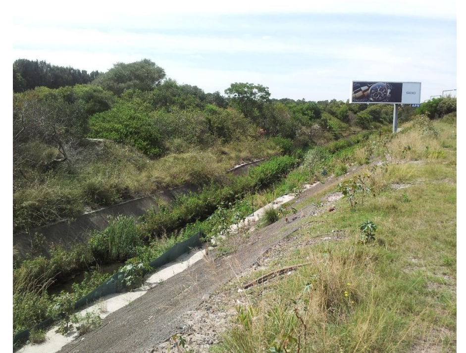
Photograph 6 – Drainage Channel that bisects the area
