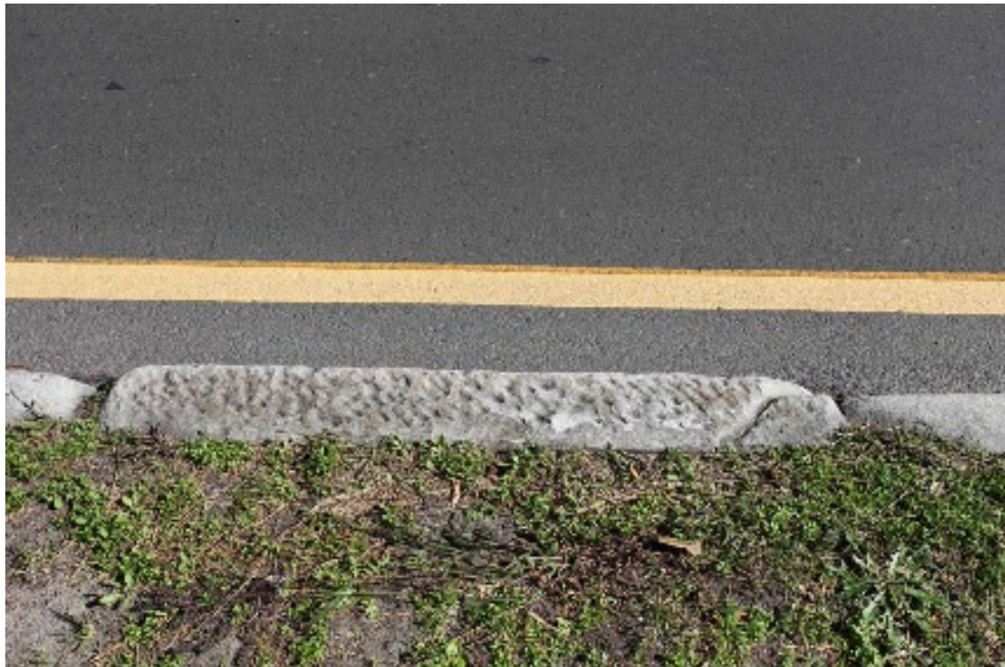
Photo 7-5 Example of sandstone kerb along Botany Road near McBurney Avenue
