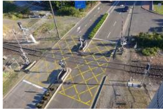
Photo 2-2 The level crossing at General Holmes Drive (facing west)
