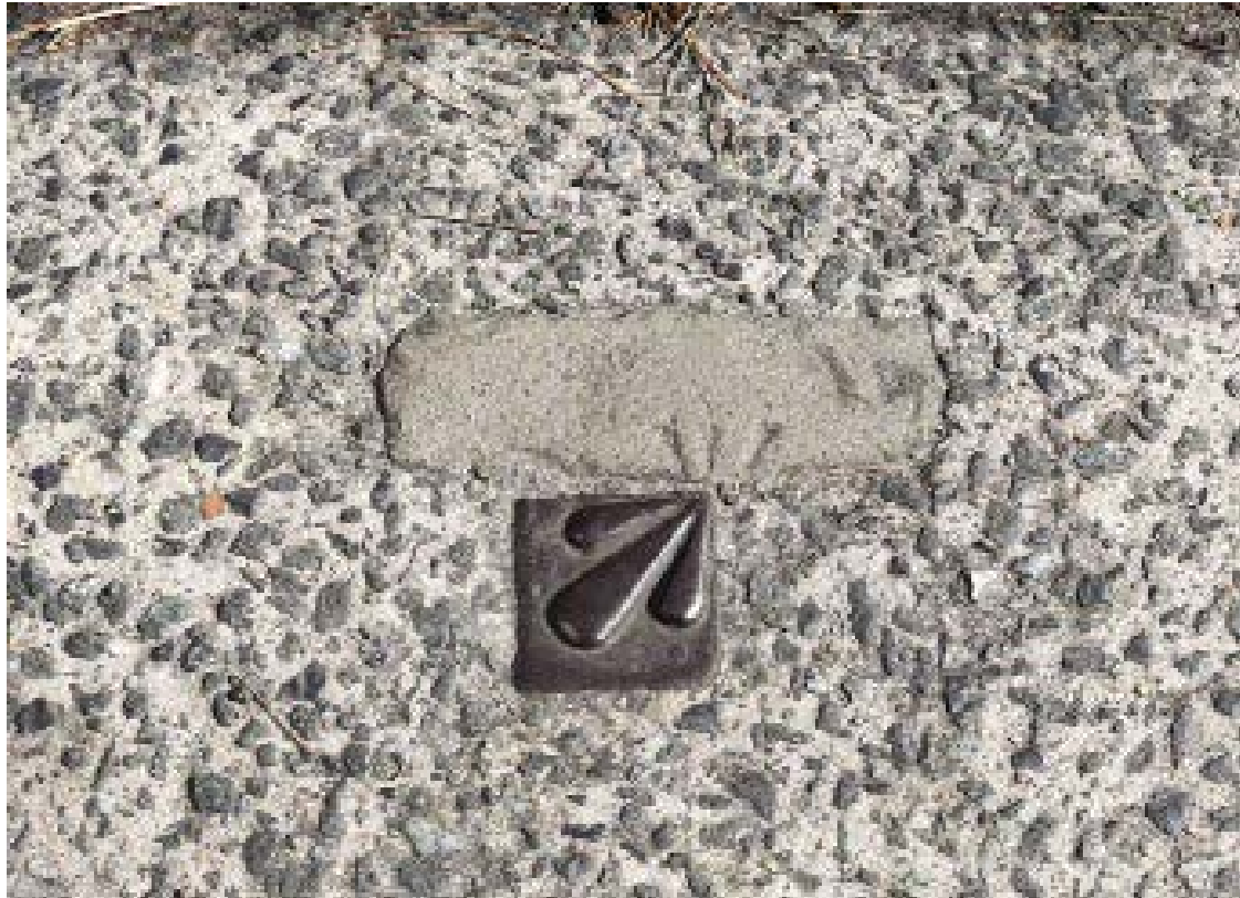
Photo 7-6 Alignment pin on sandstone kerb at McBurney Avenue and Botany Road
