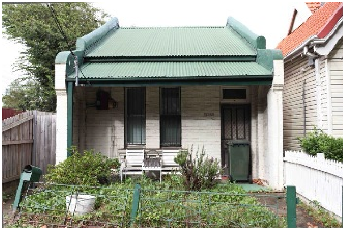
Photo 7-1 Georgian style house at 1289 Botany Road
