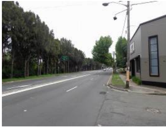
Photo 2-7 Botany Road (facing north)
