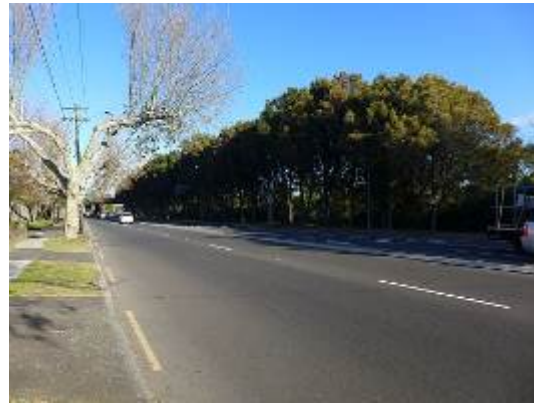
Photo 2-8 Botany Road (facing south)
