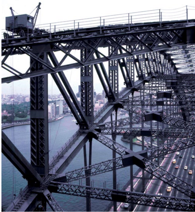
Existing arch maintenance unit on top of the Sydney Harbour Bridge arch
