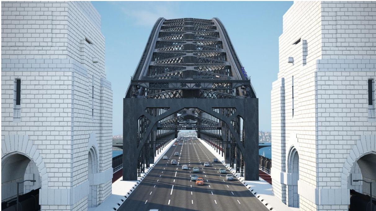
Figure 46: Render of end on view of proposed AMUs in non-operational 'park' mode. (Source: Manntech)
