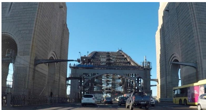
View heading north from the bridge carriageway
