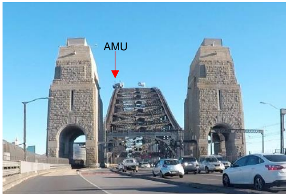
Figure 36: View south towards the SHB from the Cahill Expressway (Source: DesignInc 2017)
