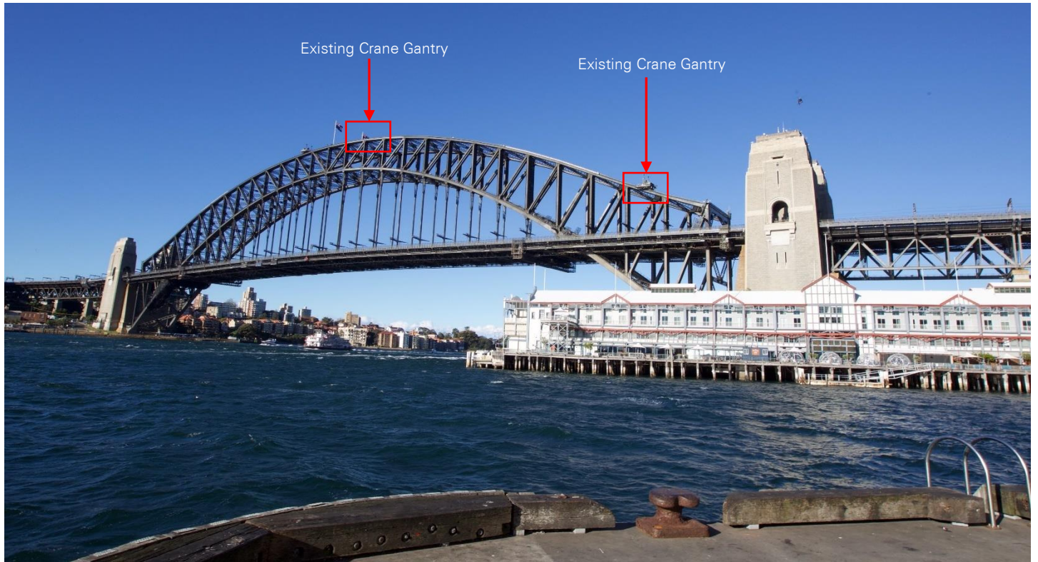
View from Pier 2/3 view, Dawes Point – Existing View
