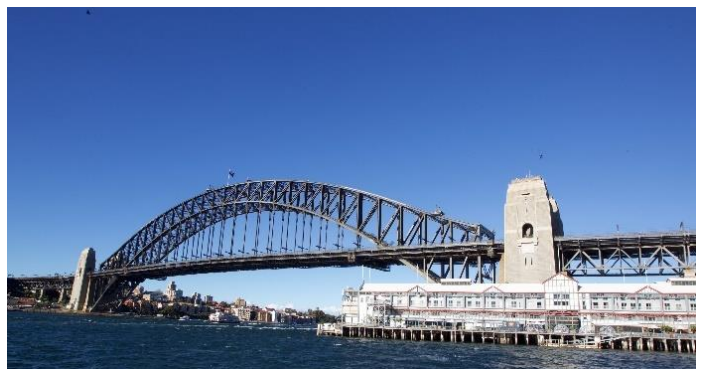
View from Pier 2/3 Dawes Point
