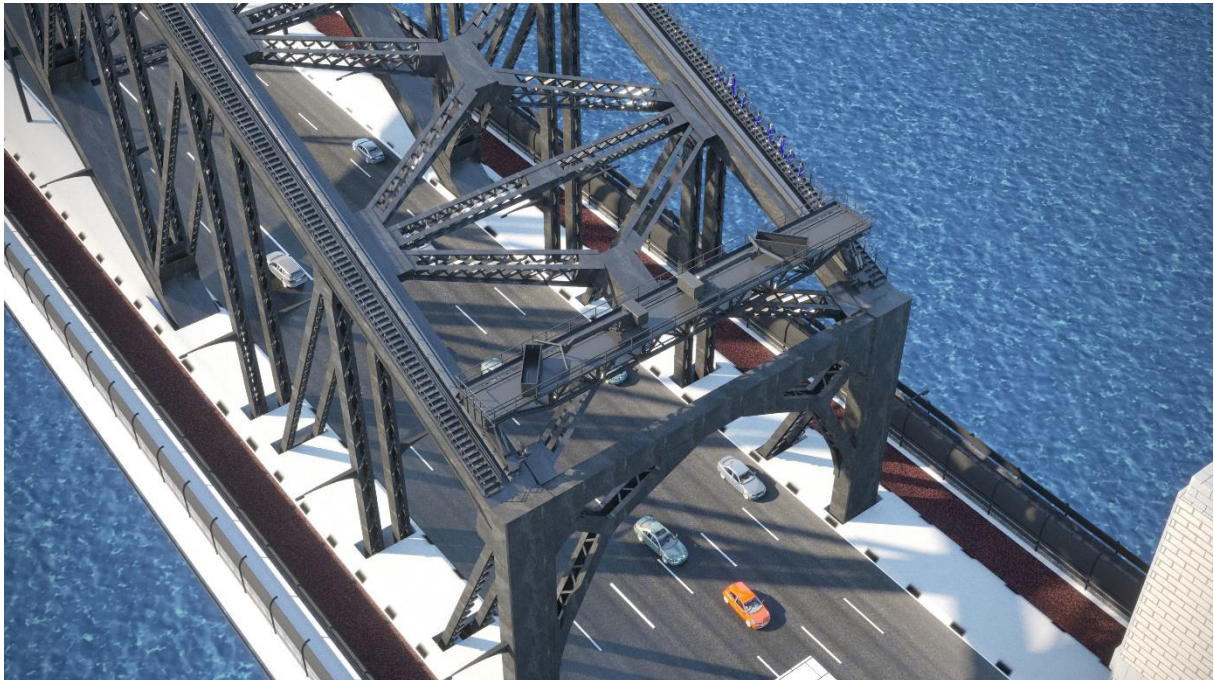
Figure 48: Render of overhead view of proposed AMUs in non-operational 'park' mode. (Source: Manntech)
