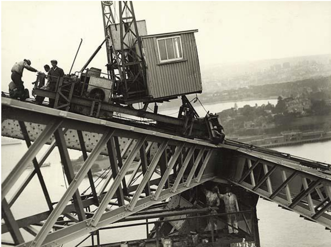
Figure 9: Historical photo showing original AMU during construction of SHB, 1931. (Source: State Records NSW. Digital ID: 12685_a007_a00704_8733000078r)
