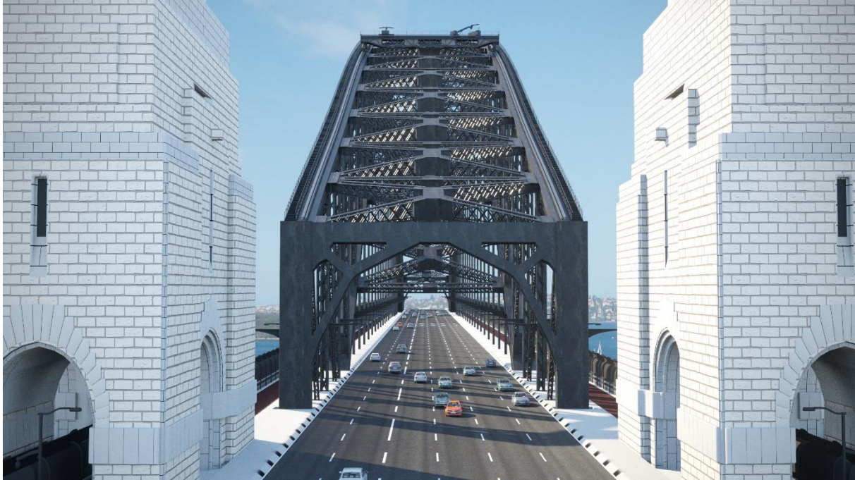
Figure 45: Render of end on view of proposed AMUs in 'operational' mode along the arch. (Source: Manntech)
