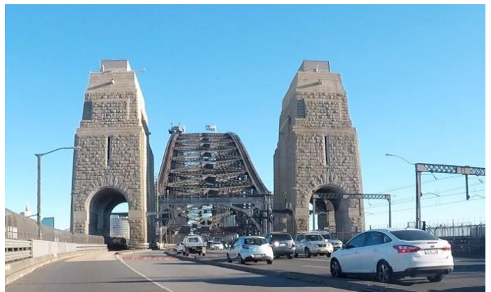
View heading south from the bridge carriageway
