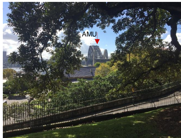
Figure 27: View north from Observatory Hill Park towards Sydney Harbour across Millers Point & Dawes Point Village Precinct (SHB seen centre).
