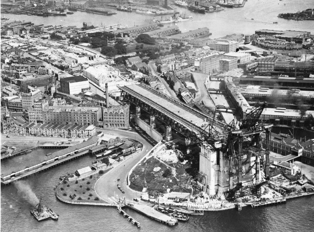
Figure 6: Aerial view of construction of the SHB and its southern approaches, c1920s. (Source: National Library Australia)
