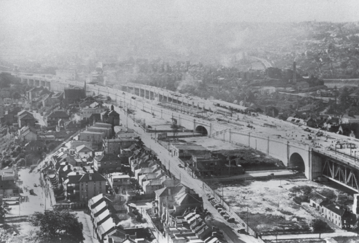
Figure 19: View of houses alongside construction of bridge approaches including arches over Fitzroy and Burton Streets, Milsons Point. 3/7/1931. Source: RTA/RMS Print 34195. Available online.
