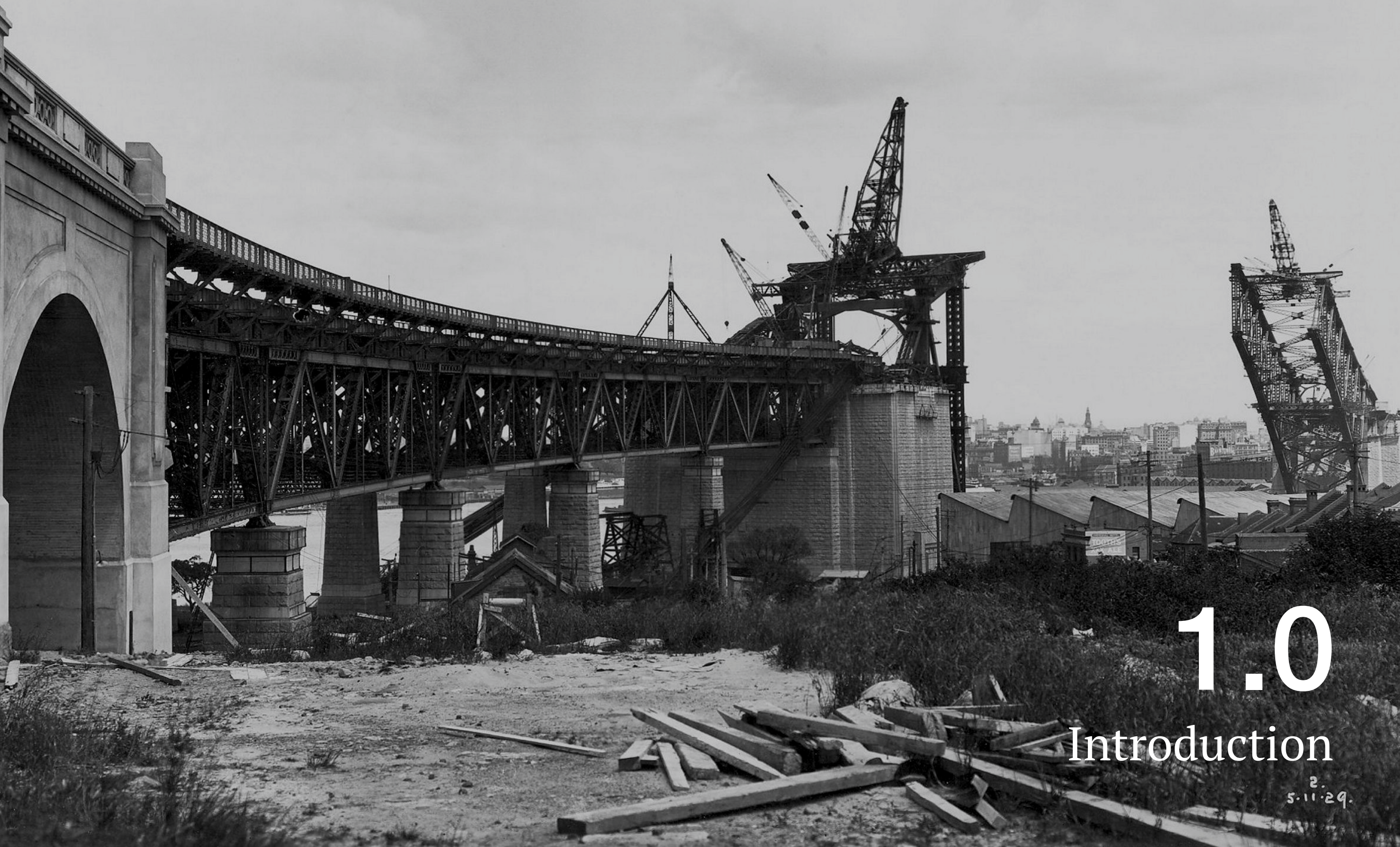
Figure 2: View south from beside the Fitzroy Street arch, Milsons Point, showing completed spans 6,7,8,9,and 10. Creeper Cranes on bridge. 5.11.1929. Source: RTA/RMS print 34479. Filename:19291105HB34479.jpg
