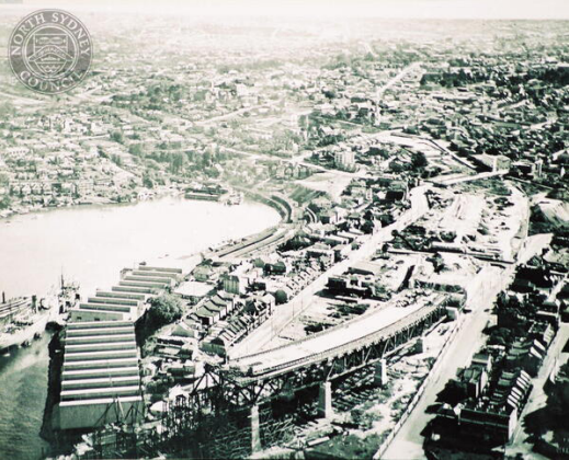
Figure 16: Aerial view of construction of Bradfield Highway approaches to Sydney Harbour Bridge, late 1920s. Source: State Rail Authority/State Records. One of set of 10 photographs showing rail/tram transport from SRA Archives, LPF 330-332 and 493-499 Available online via Stanton Library Historical Services.
