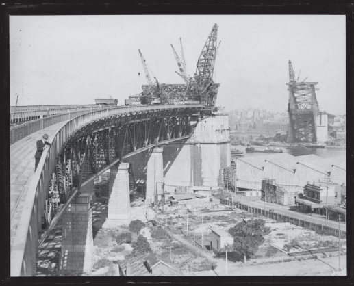
Figure 17: Cranes positioned at both sides of the unfinished Sydney Harbour Bridge, Sydney, 1929 [picture]. Source: National Library of Australia. Available online at: https://nla.gov.au/443/tarkine/nla.obj-162053201
