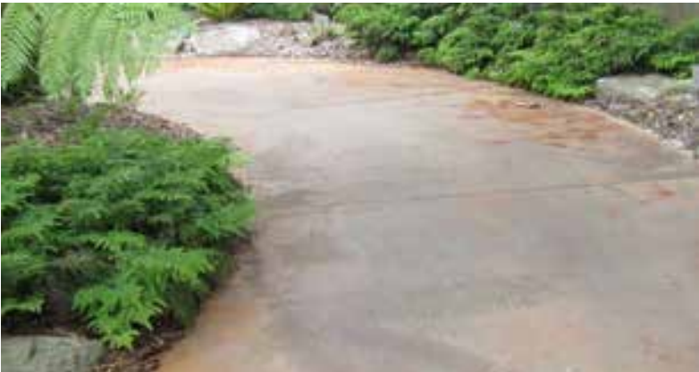
Coloured concrete with feature coloured aggregate
