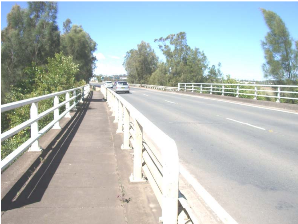
Photo 2 - Narellan Creek bridge travelling north
