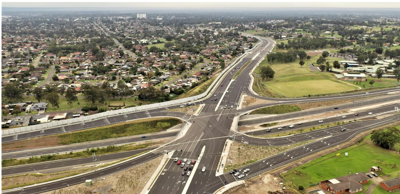
The Northern Road and M4 Motorway interchange (looking north)
