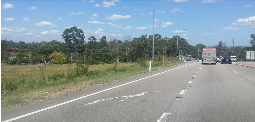
Figure 6-2: Current view east along The Northern Road facing South
