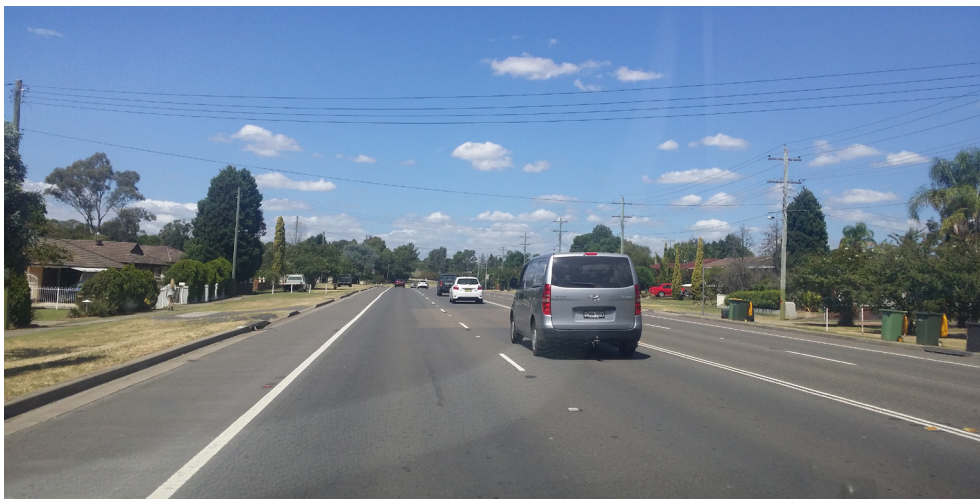
Figure 6-8: Current view of The Northern Road facing south at approach to Bringelly Road
