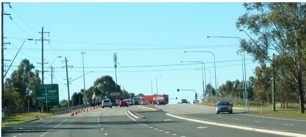
Figure 6-5: Current view of north bound approach to the interchange
