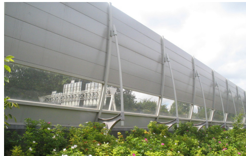
Figure 8-2: (above left) An example of how transparent noise walls and throw screens can be integrated in a refined structure (source: http://www.npkdesign.com/wp-content/uploads/2014/07/2150-Adam-geluidsscherm-1.jpg )
