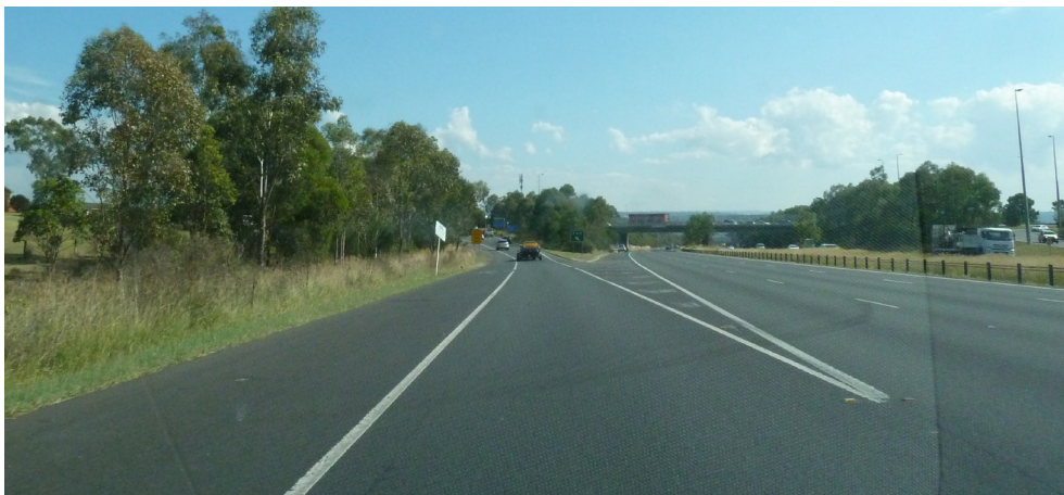
Figure 6-4: Current view of west bound off ramp, M4 Motorway
