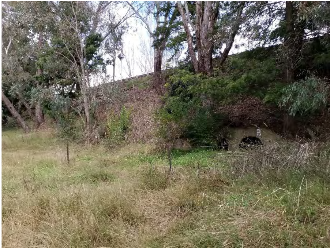
Figure 3-5 Dam within the proposal area
