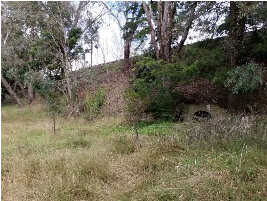
Figure 3-6 Culvert under the Snowy Mountains Highway
