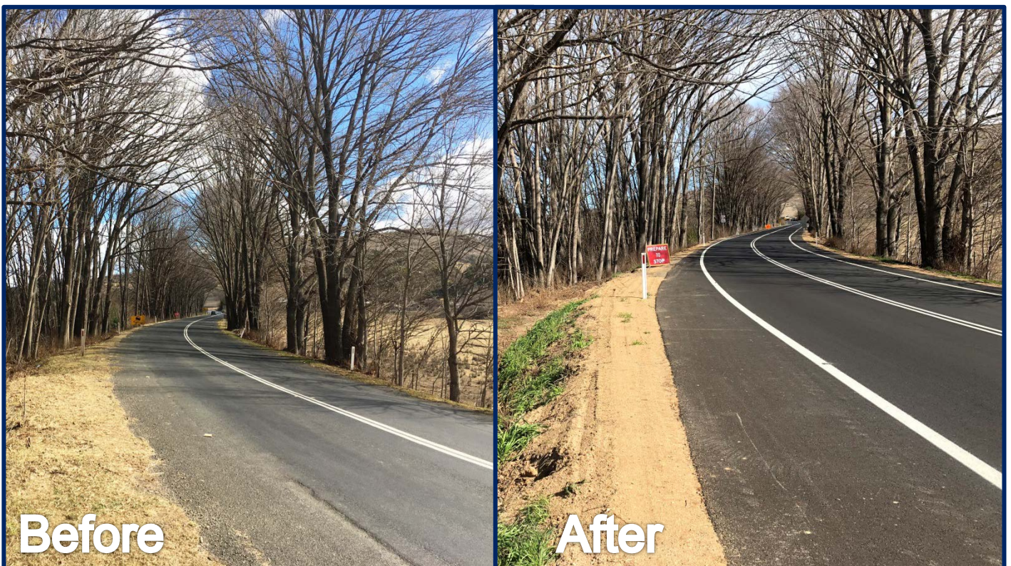
Vale Road, north of Perthville, before and after upgrade work.
