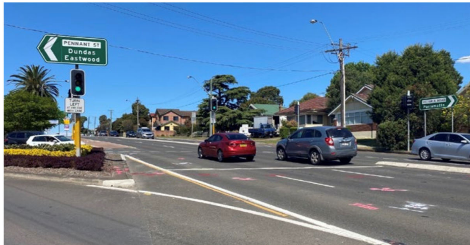
Intersection of Victoria Road and Pennant Street, Parramatta
