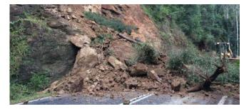
The road through the Gordonville Cutting area has been included in the work to remove vegetation, scaling of loose rocks and boulders.
