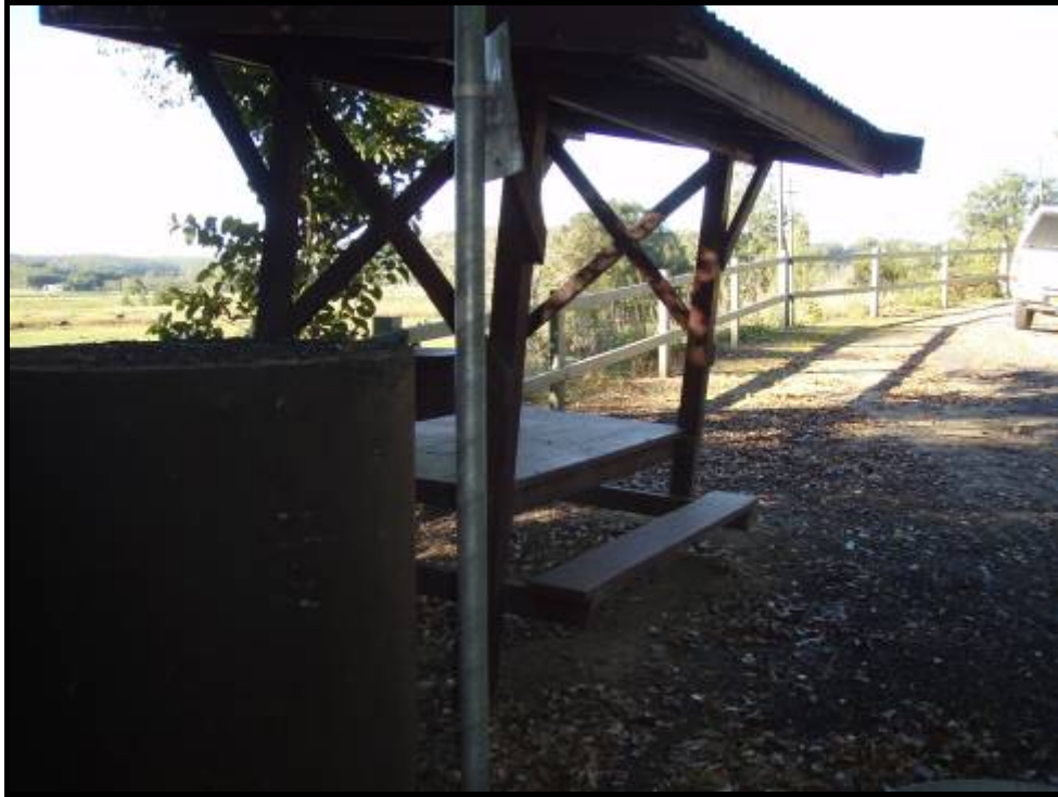
Photo: Mount Lookout visitor facilities (Image: SDW)
