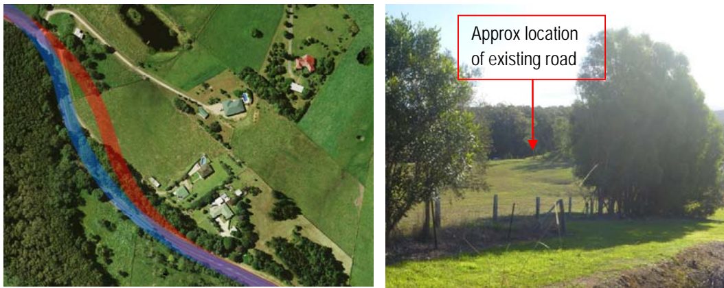
Plate 3.9 Viewpoint 5 – Aerial (Option A = Blue; Option B = Red) and a Typical View Experienced Near Dwelling
