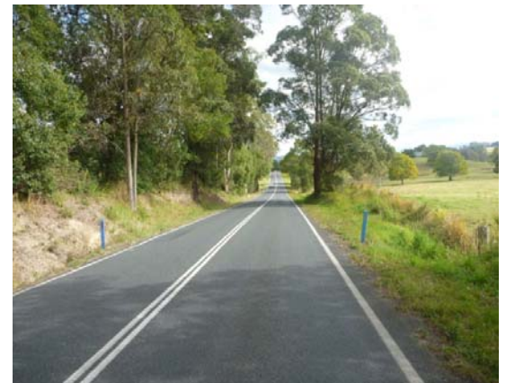
Plate 1.6 View West along Waterfall Way - Approx 2.8km West of Pacific Highway
