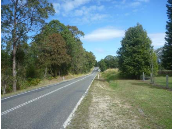
Plate 1.1 View West Along Waterfall Way - Approx 850m West of Pacific Highway
