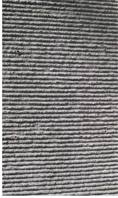
In situ concrete with a rope finish
