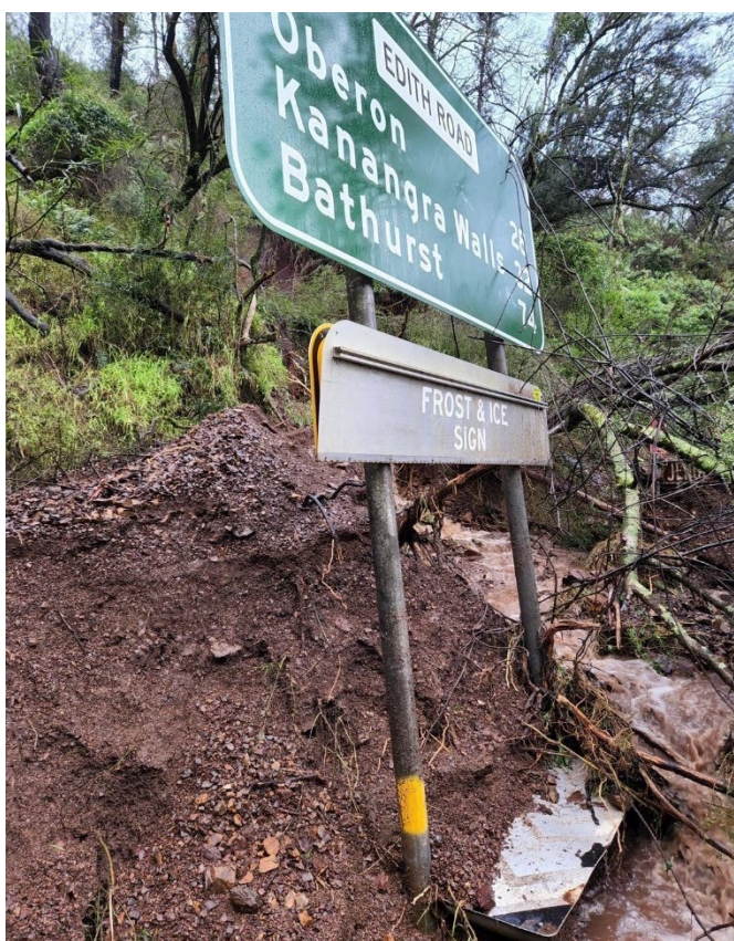
Debris following excessive rain in July
