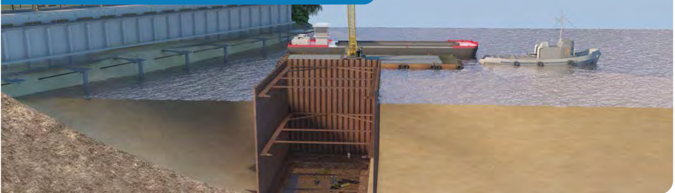
Artist's impression of cofferdam construction in Sydney Harbour
