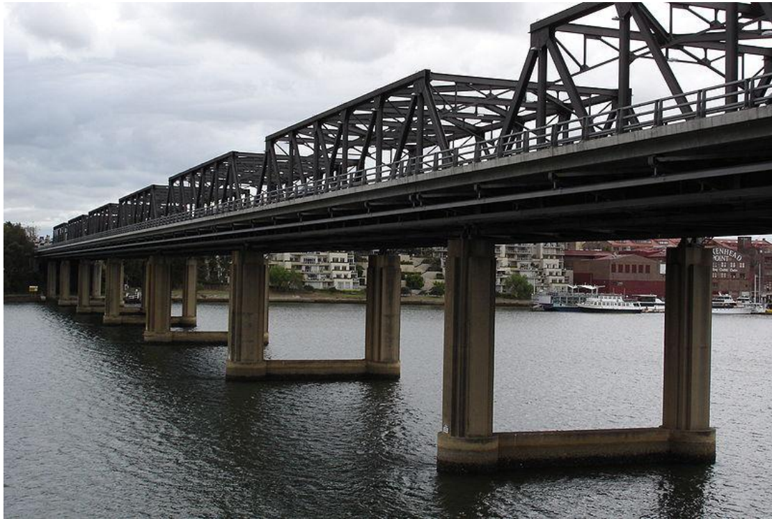
Figure 4-8 Example of a truss bridge (Iron Cove Bridge, Sydney)
