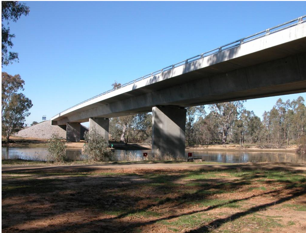
Figure 4-4 Example of an incrementally launched bridge (Corowa, NSW)
