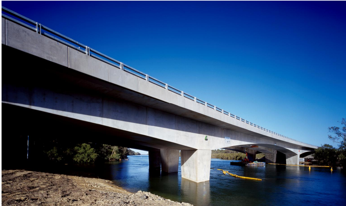
Figure 4-5 Example of an in situ balanced cantilever bridge (Brunswick, NSW)
