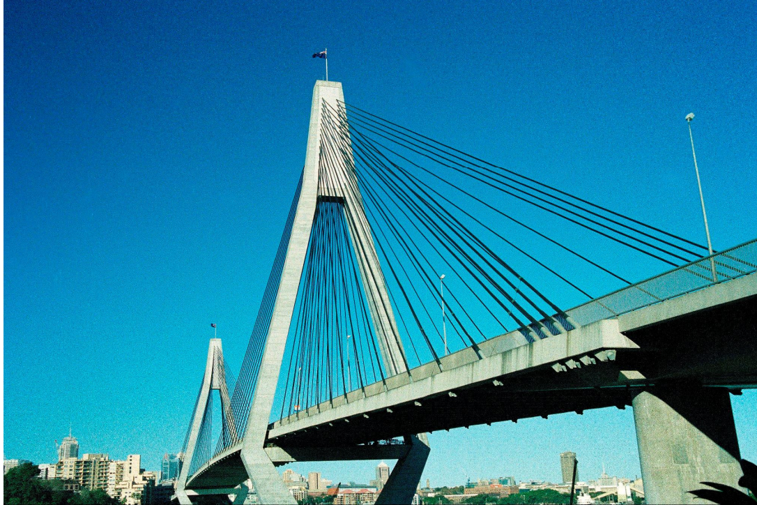
Figure 4-9 Example of a cable stayed bridge (ANZAC Bridge, Sydney)
