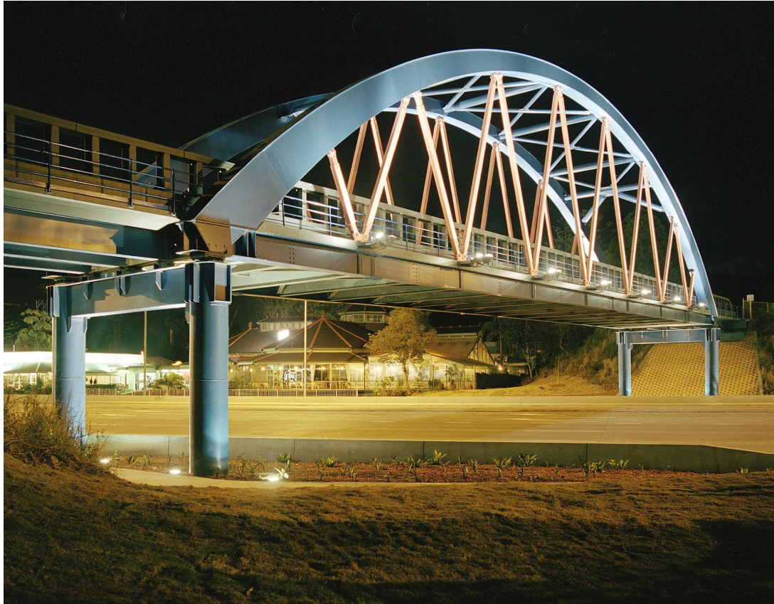
Figure 4-7 Example of an arch bridge with arch above deck (Coffs Harbour, NSW)
