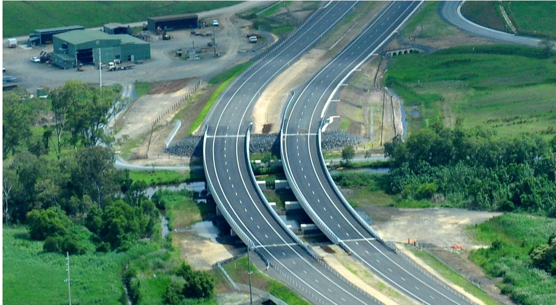
Figure 4-10 Example of a cast in-situ bridge (Emigrant Creek, Sydney)
