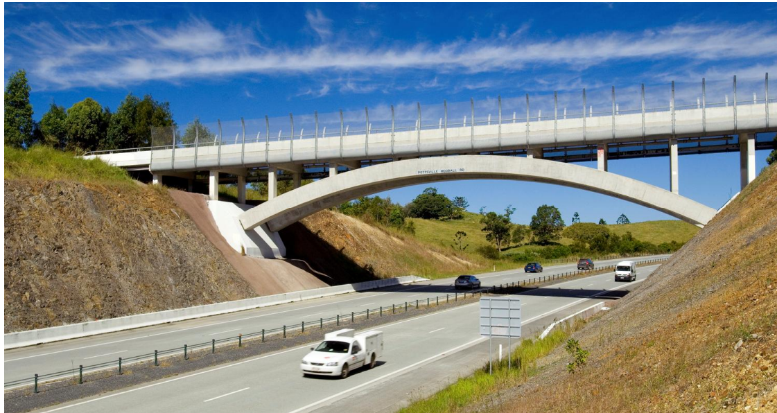
Figure 4-6 Example of an Arch Bridge with arch under deck (Yelgun, NSW)
