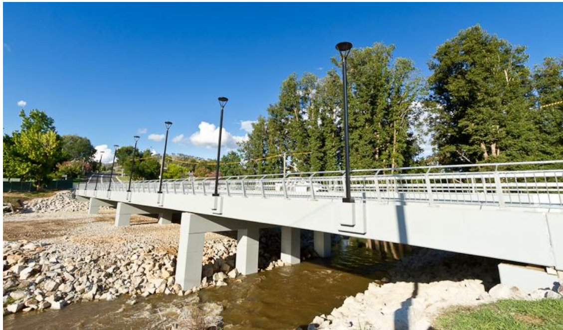
Figure 4-3 Example of a precast concrete plank bridge (Adelong Bridge, NSW)
