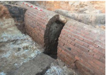
Brick barrel drain (showing 1930s sewer work damage) to be preserved in its current location
