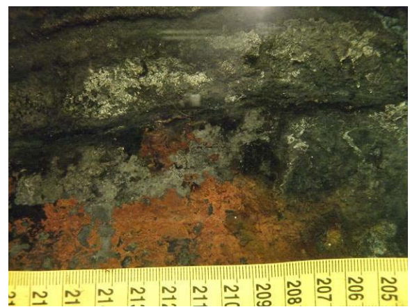
Circumferential crack on column 5U
