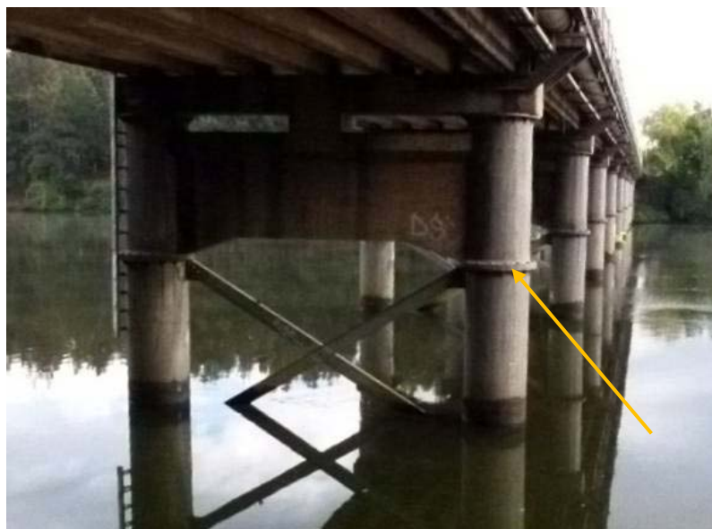
View of above water part of bridge pier showing lower flange used as reference level for recording height on piers
