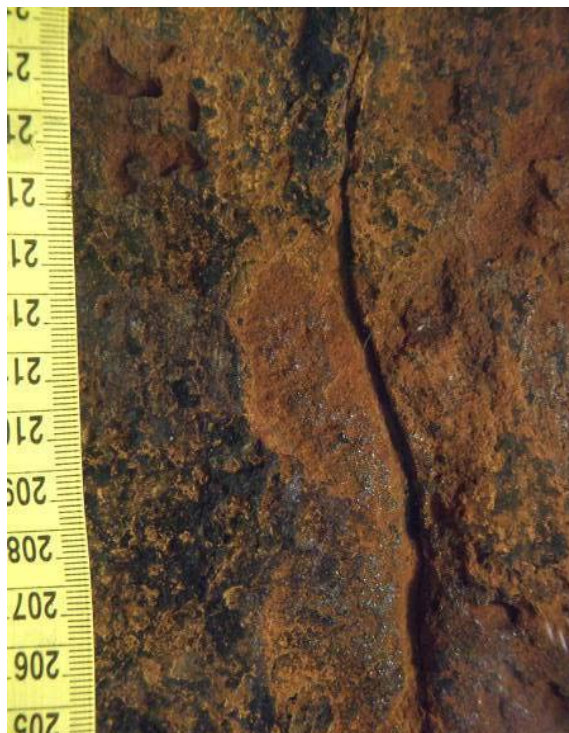
Vertical crack on column 5U on downstream side, estimated to be > 2 mm wide at its base
