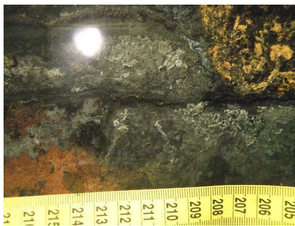
Circumferential crack on column 5U
