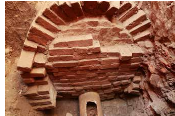
Images showing the exposed barrel drain and associated box drains in-situ within Thompson Square during archaeological excavations in 2018. RMS.
