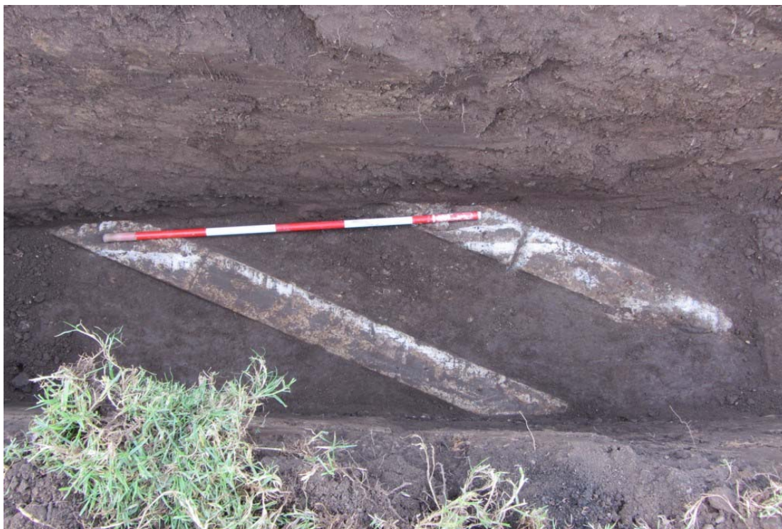
Plate 117: View east showing concrete beam in Test Pit 5 laid as part of the work in 1894 to improve the approaches to the bridge after it had been raised in height], scale 200 millimetre increments.
